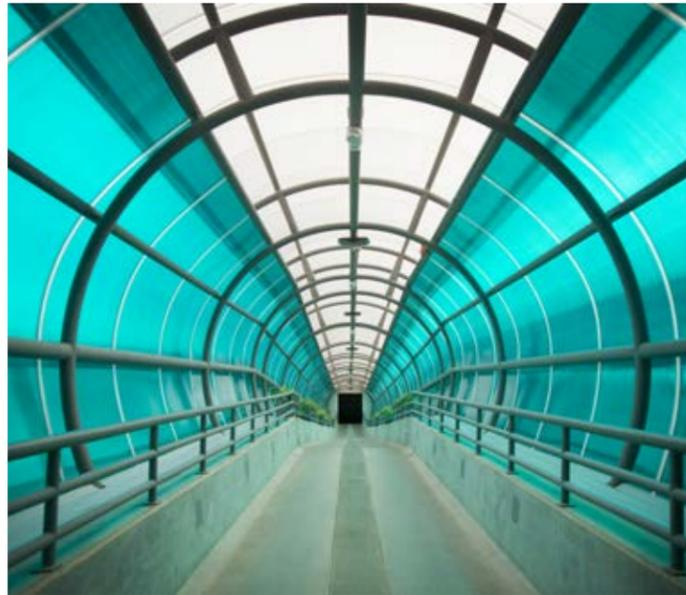
High light transmission combined with thermal insulation from the multiwall structure makes Marlon ST an ideal material for rooflights and vertical glazing. Natural light and U-values as low as 0.83W/m<sup>2</sup>K contribute to a more energy efficient building whilst the attractive appearance of the sheet enhances design capabilities for a stunning architectural feature.
