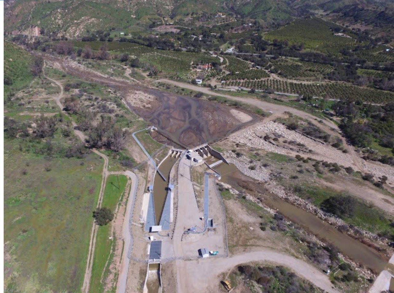
Robles Diversion and Fish Passage Facility 2019
