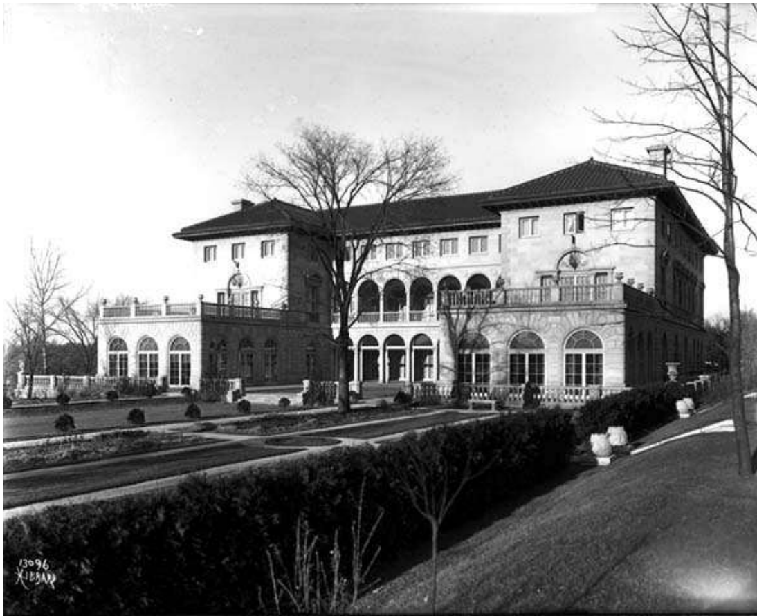
Rear façade of the Lake of the Isles mansion. Its scale reflected Charles Gates' intention to create a residence capable of accommodating both family life and an extraordinary art collection.
