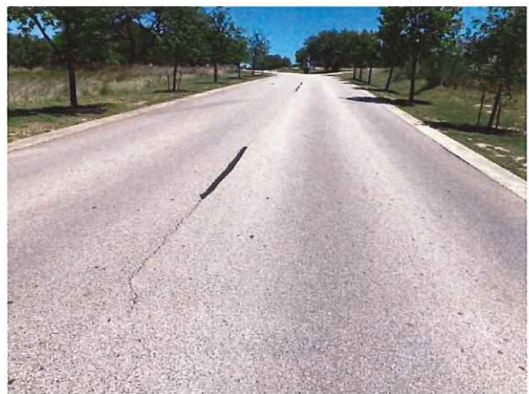
Asphalt pavement street overview
