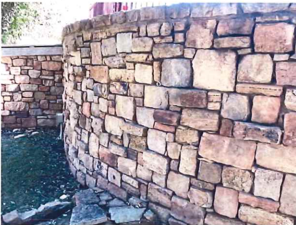
Masonry retaining wall
