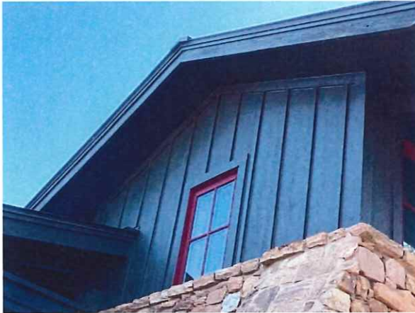
Fiber cement siding
