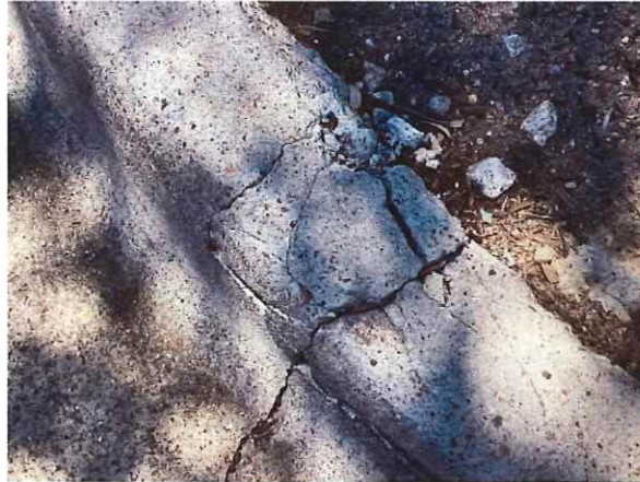
Concrete spalls
