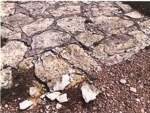
Masonry deterioration
