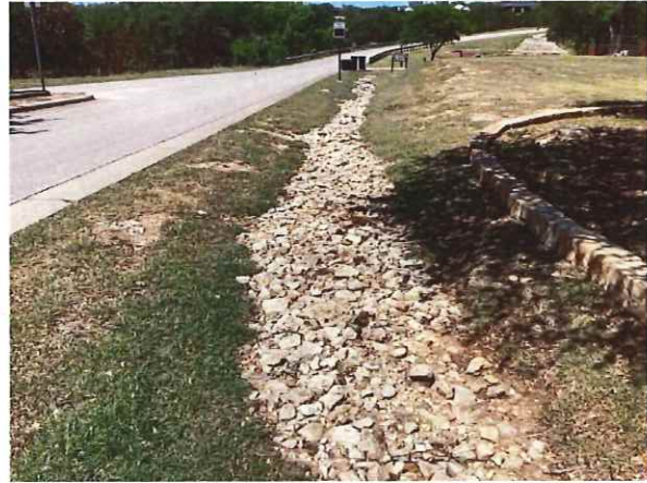
Rip rap along drainage swale
