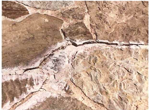
Mortar deterioration
