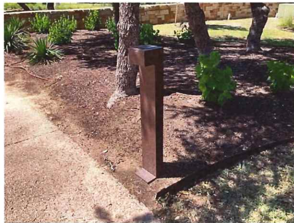
Bollard light fixture
