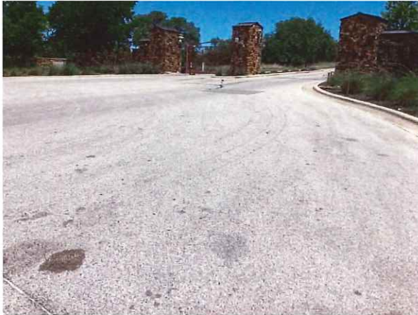
Asphalt pavement street overview
