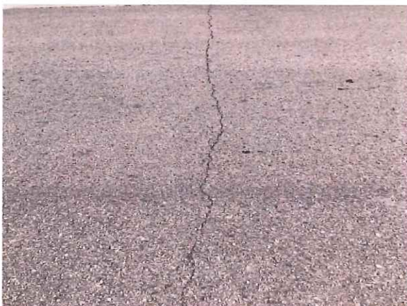
Pavement cracks
