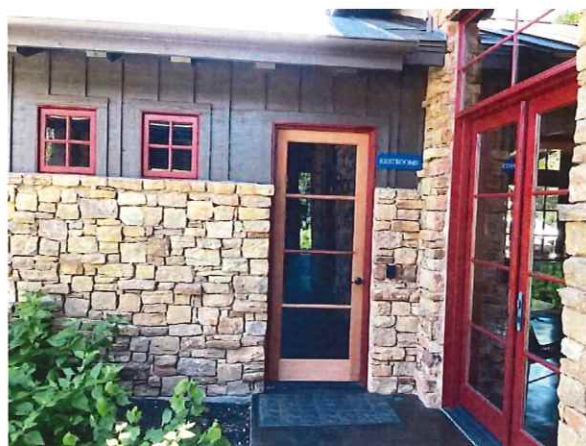
Windows and doors
