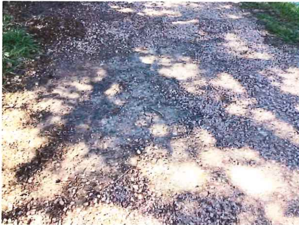
Area lacking granite coverage
