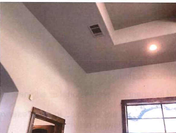
Paint finishes in good condition
