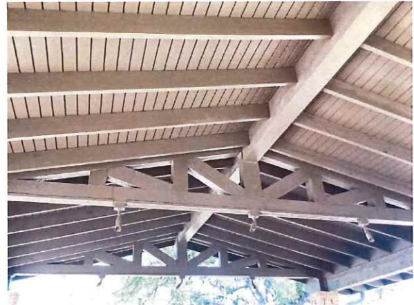
Wood soffit and trim at the mailbox kiosk
