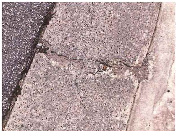
Concrete cracks
