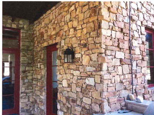
Exterior masonry walls
