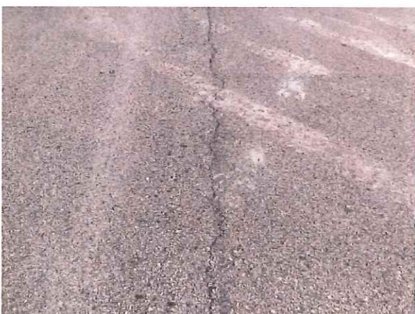
Pavement cracks
