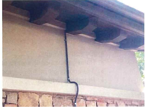
Exterior stucco walls
