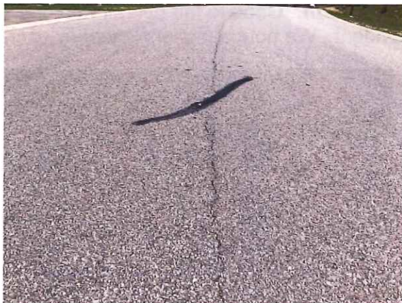
Centerline cracks
