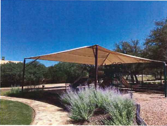
Shade structure at the playground
