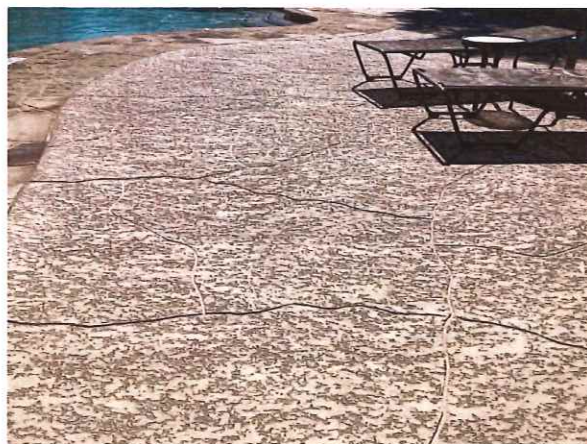
Textured coating in good condition
