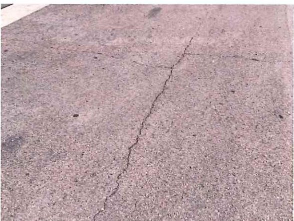
Pavement cracks
