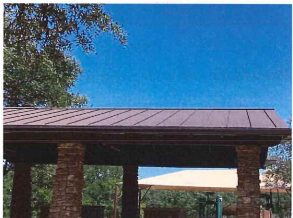
Metal roof at the mailbox kiosk
