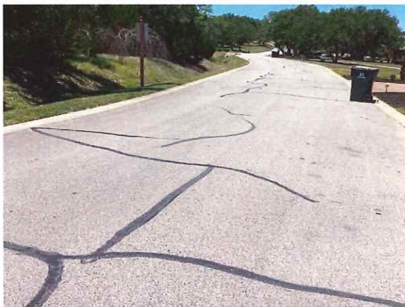
Previous crack repairs
