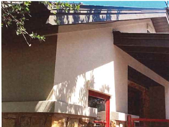
Exterior stucco finish
