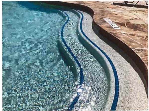
Pool plaster and tile finishes
