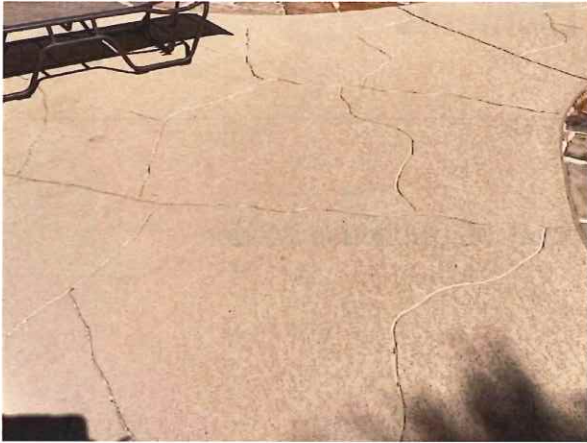
Coated concrete pool deck
