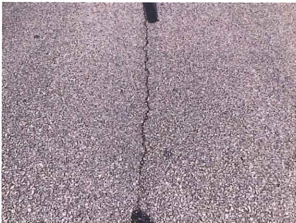
Pavement cracks
