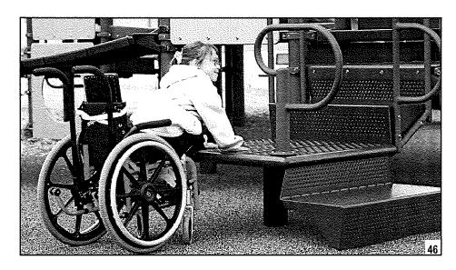
A transfer system typically consists of a transfer platform, transfer steps, and transfer supports.
