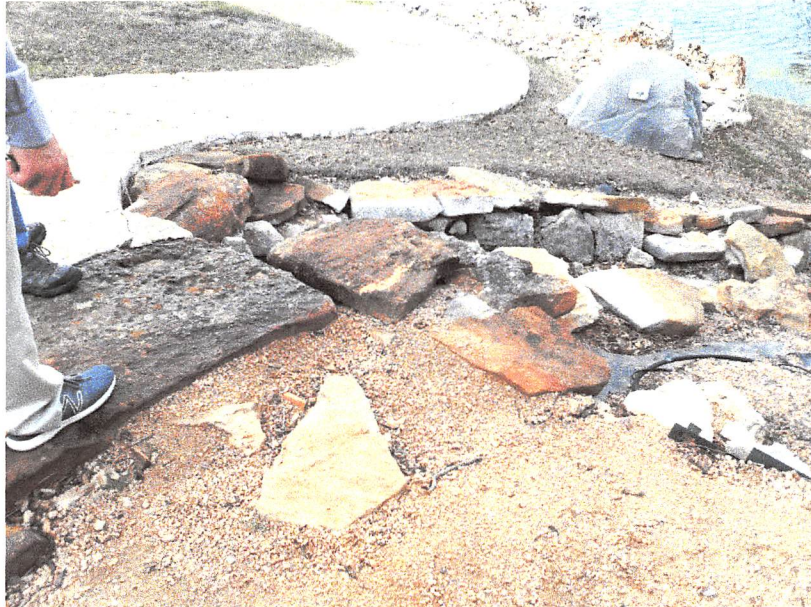
Drainage Feature Repair Lower Pond Trail to Lower Pond
