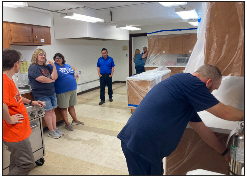
Plastic was taped to the walls and cabinets to keep the dust out during the flooring work.
