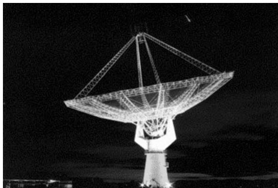
Fig. 4 One of the thirty telescopes of the GMRT (Giant Metrewave Radio Telescope) near Pune in India. This giant radio telescope was conceived and built by Govind Swarup and his colleagues at the Tata Institute of Fundamental Research in Mumbai
