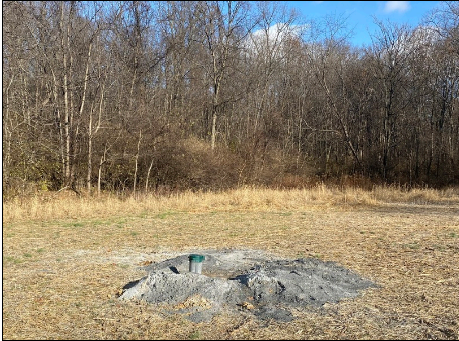
3 - Monitoring well PZ01.
