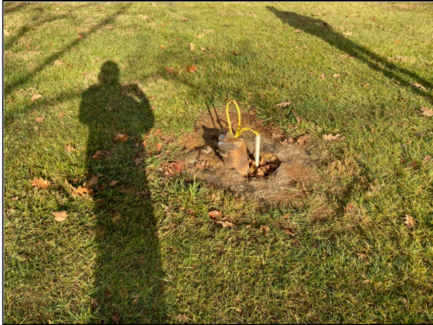
1 - Unused well at 3497 Ritner Highway.
