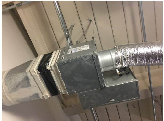
Photograph 4 – Flex Duct at TU Inlet
