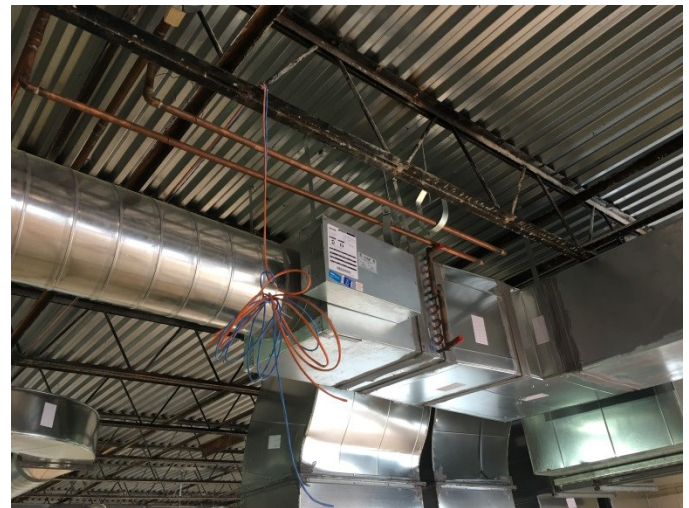
Photograph 6 – Hard Duct Extension at TU Inlet
