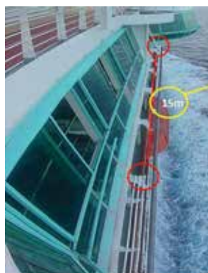
15m section with no dedicated catwalk or secure anchor rail
