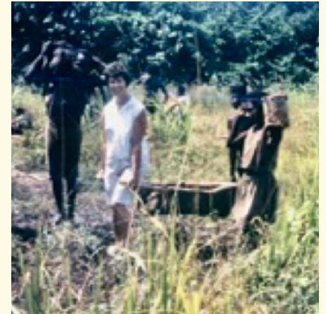
Repairing the airstrip with jungle "wheelbarrow"
