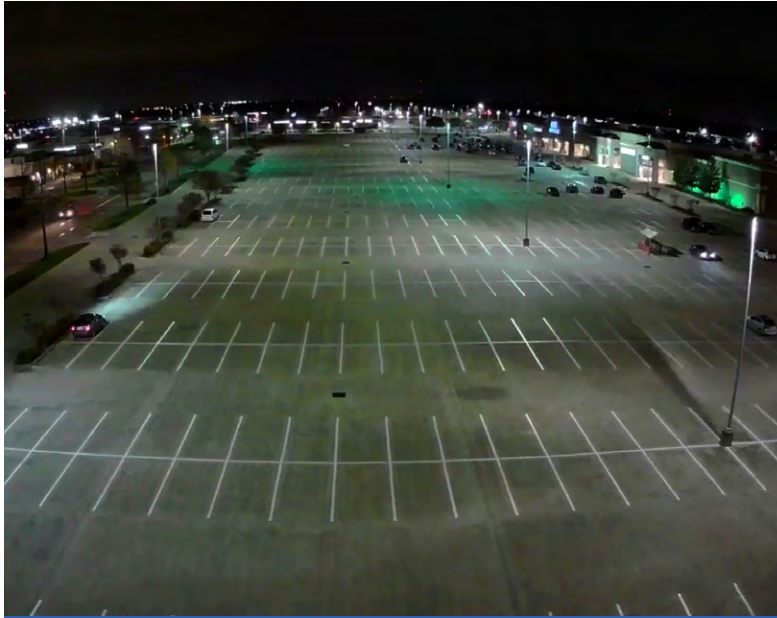
BEFORE: OUTDATED PARKING LOT LIGHTING
