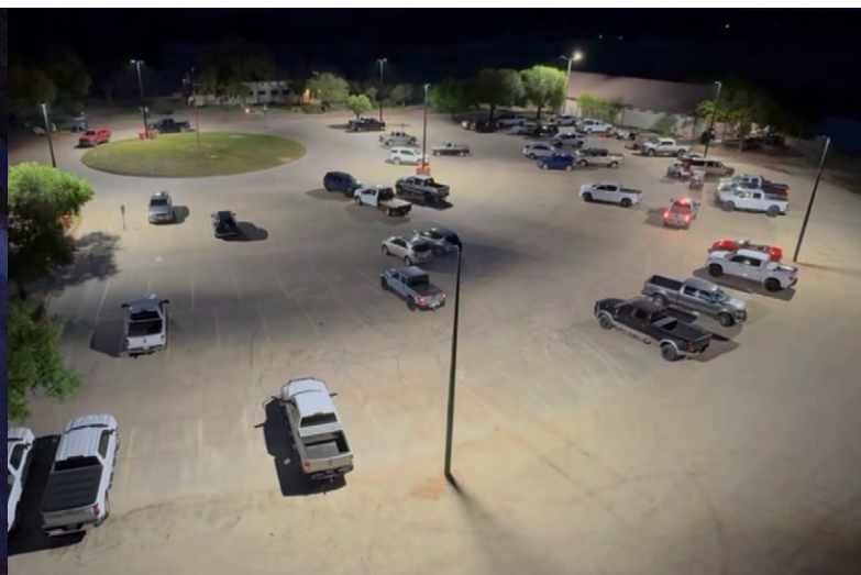
AFTER: NEW LED PARKING LOT LIGHTING
