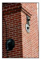
Anchor plates for reinforcing rods are visible in several places on the exterior of the old section of the church. Those include the corners at the front of the structure and the spaces immediately above the three northerly windows on each side.
