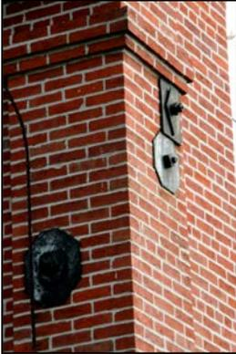
Anchor plates for reinforcing rods are visible in several places on the exterior of the old section of the church. Those include the corners at the front of the structure and the spaces immediately above the three northerly windows on each side.
