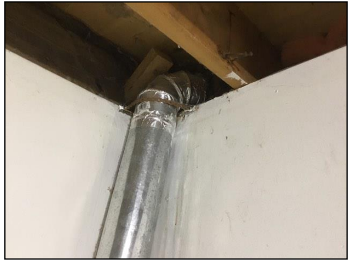
77. Clothes dryer vented to exterior
