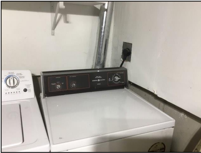
76. Clothes dryer vented to exterior
