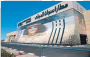
■ Airport, Assuan, Egypt
