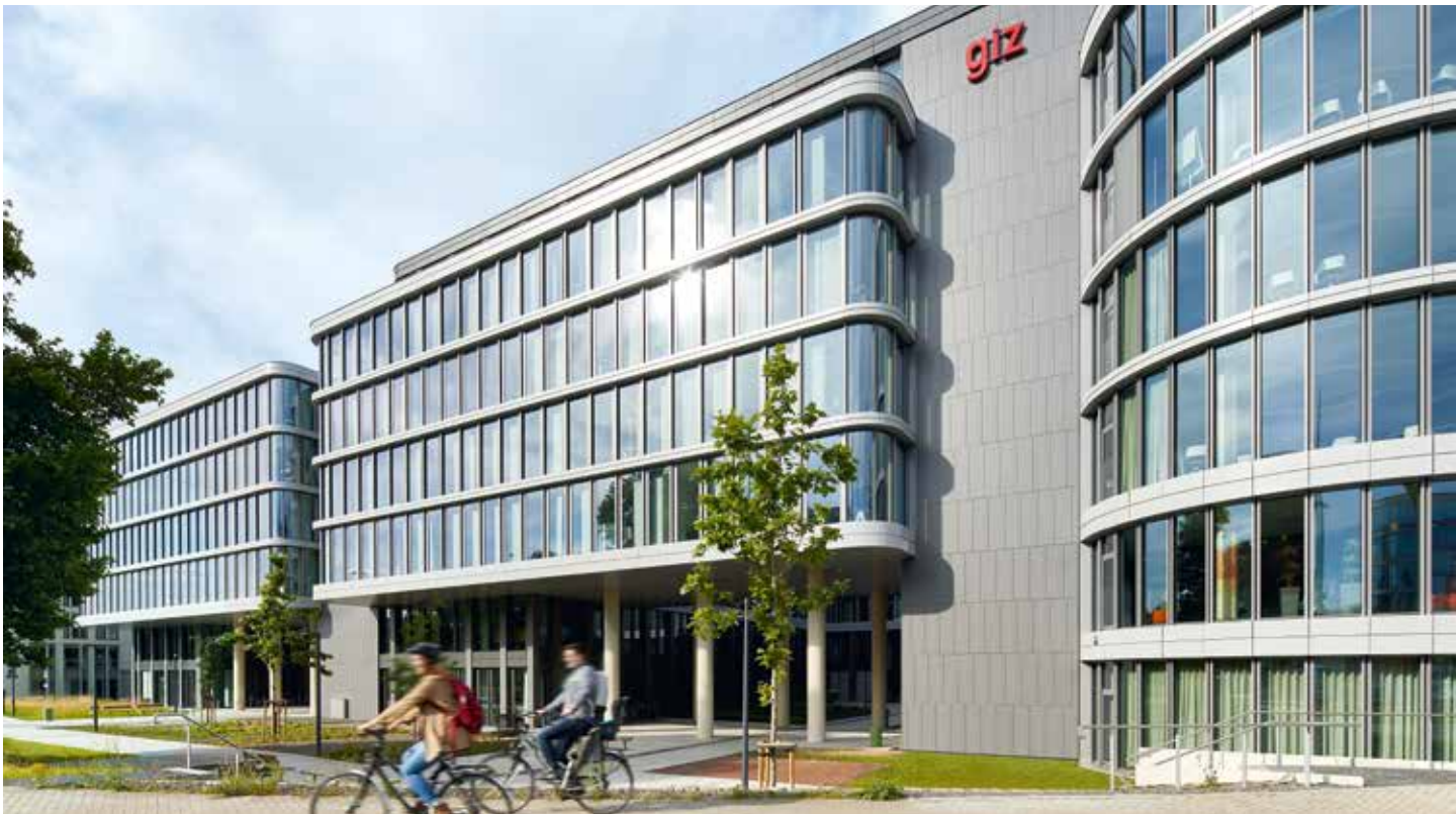
GIZ-Campus, Bonn, Germany / Architect: CLP GmbH, Koblenz / Year: 2019 / Photo: Jochen Stüber
