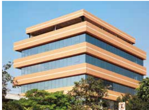
Jurubatuba Building, Sao Paulo, Brazil Architects: alériaTaurino, Sao Paulo/SP, Brazil
