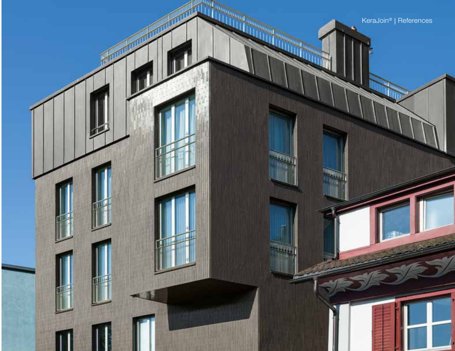
Residential and commercial building Badstraße, Switzerland / Architects: Schoop Architekten AG, Baden, Switzerland / Year: 2014 / Products: Craft Photo: Adriano Faragulo
