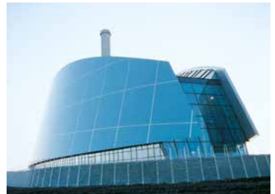
Thermal power station, Viborg, Denmark / Architect: Arkitekterne, Peter Kjelgaard & Thomas Pedersen M.A.A., Viborg
