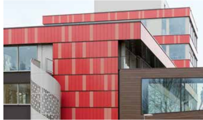
Administrative building, Groningen, the Netherlands / Architect: SKETS architectuurstudio / Year: 2015 / Photo: Marcel van der Burg
