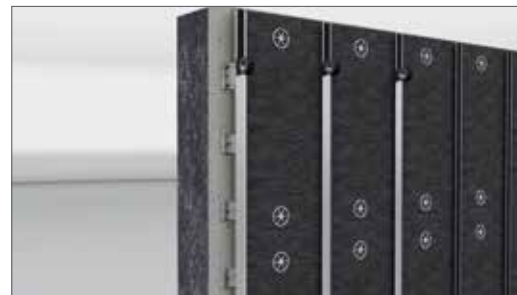
Apply joint tape on vertical bearing profiles
