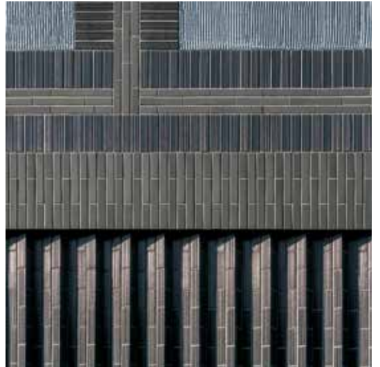
Apartment building Leopold, Sursee, Switzerland Architect: GKS Architekten Generalplaner AG / Year: 2018 Products: Craft / Photos: Adriano Faragulo
