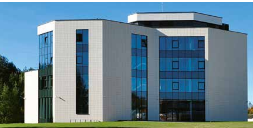
Riomer University, Vilnius, Lithuania / Architect: Arch. Irmantas Gudavičius Statybos projektu valdymas / Year: 2015 Photo: Nedas Bobinas, cb-products
