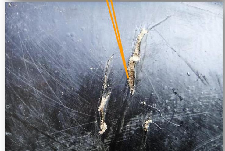
The excavated pit made at the location of the isolation cover damage, detected according to the results of the contactless inspection.
