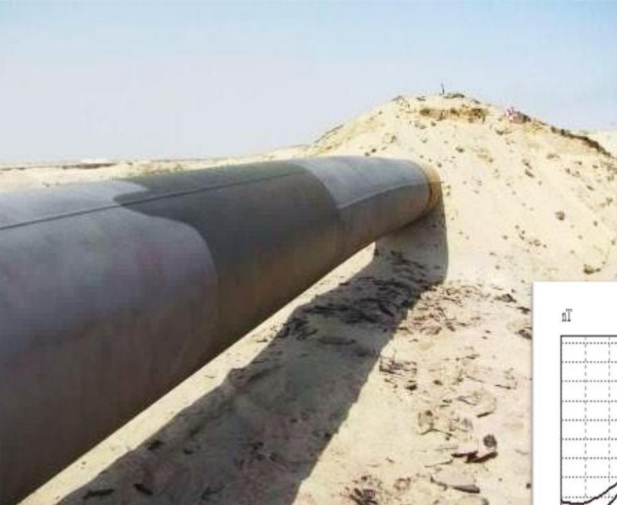
The magnetogram of changing of the full vector of magnetic induction shows significant stress (bending moment), caused by curving of the pipeline due to the pressure of sand. ILI made a few months before defined the pipeline as “no problems”.
