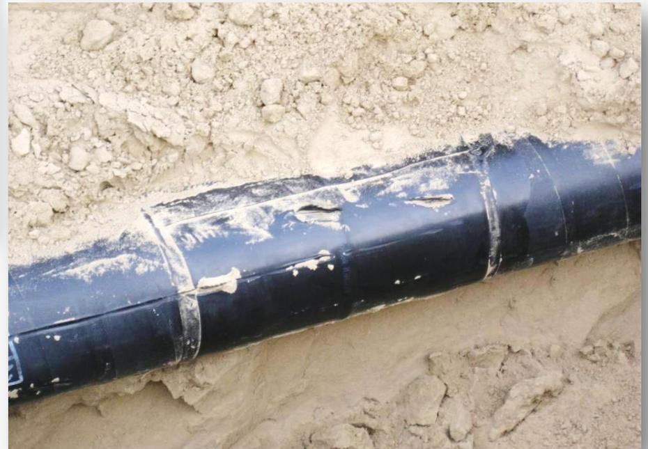
The excavated pit, made at the location of the magnetic anomaly the concentrator of the tensions (repair construction) was found.
