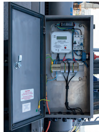
Figure 11. The Webserver Monitoring cabinet
