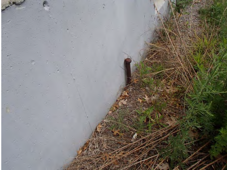
GEC Project No. 1936-0010. June 12, 2020. 2210 Providence Highway, Walpole, MA. View of the UST vent pipe protruding from the ground along the south exterior wall of the Site building prior to excavation
