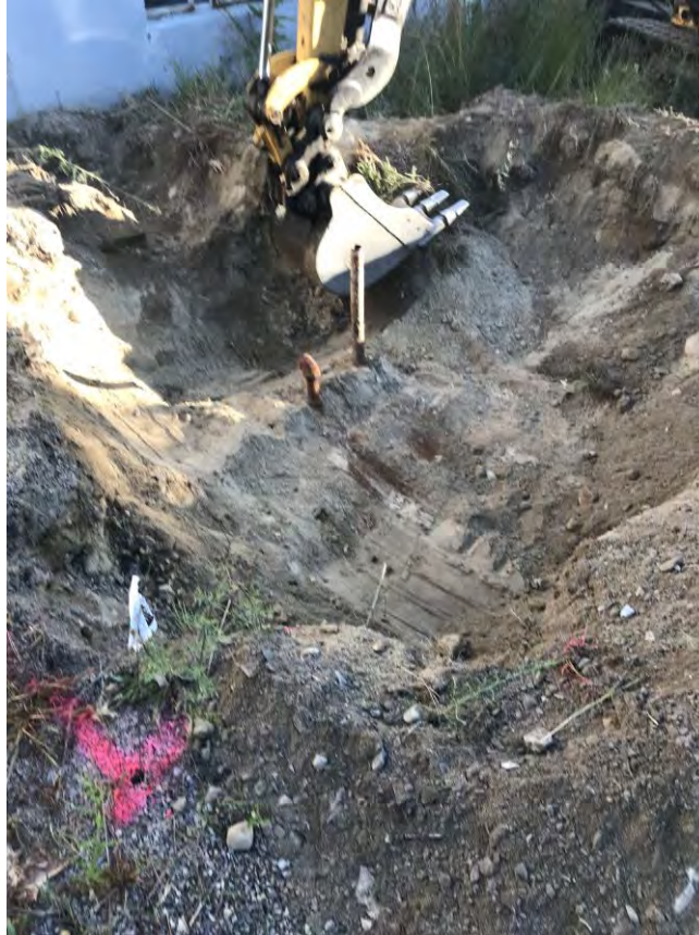
GEC Project No. 1936-0030. July 30, 2020. 2210 Providence Highway, Walpole, MA. Photograph of the uncovering of UST.
