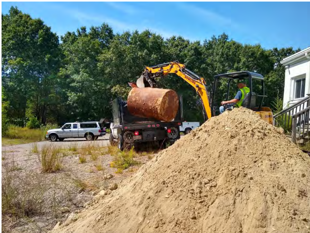
GEC Project No. 1936-0030. July 30, 2020. 2210 Providence Highway, Walpole, MA. General view of the tank being placed on the truck for off-Site disposal.
