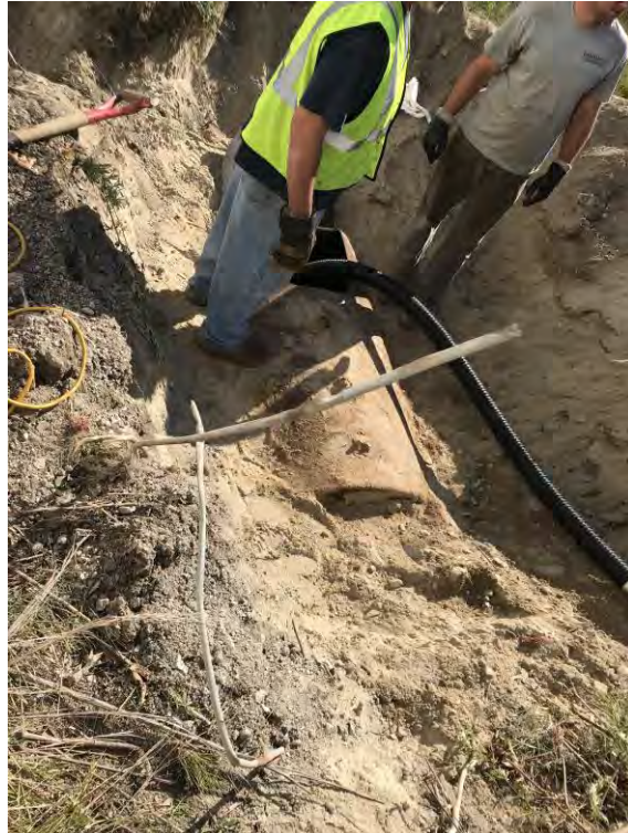
GEC Project No. 1936-0030. June 12, 2020. 2210 Providence Highway, Walpole, MA. View of the residual oil/water mixture being pumped out from the UST.
