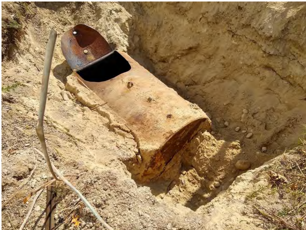
GEC Project No. 1936-0030. July 30, 2020. 2210 Providence Highway, Walpole, MA. Photograph of the exposed UST and soil conditions along its south and east sides.
