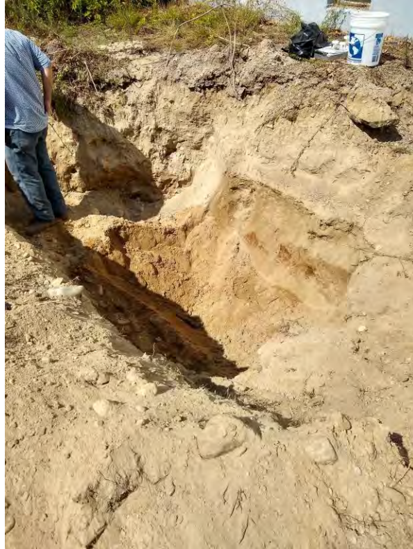
GEC Project No. 1936-0030. July 30, 2020. 2210 Providence Highway, Walpole, MA. General view of the soil conditions in the tank grave following removal of the UST.
