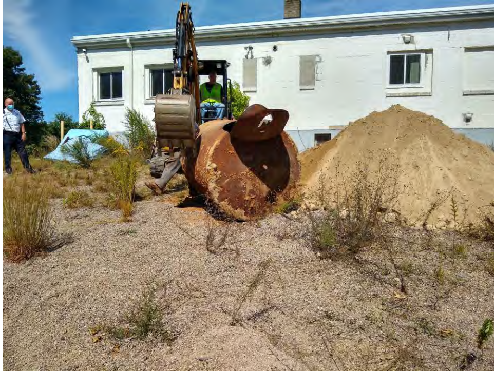
GEC Project No. 1936-0030. June 12, 2020. 2210 Providence Highway, Walpole, MA. View of the UST being pulled out from the ground under the witness of the Dire Department.
