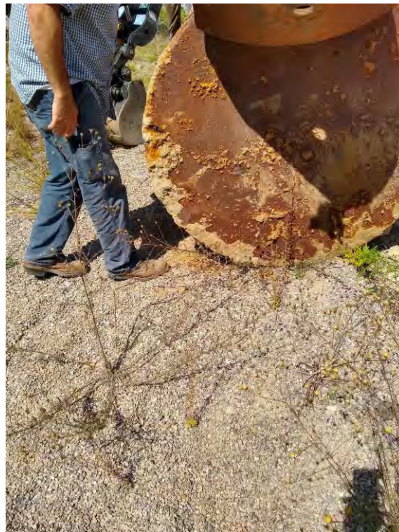
GEC Project No. 1936-0030. June 12, 2020. 2210 Providence Highway, Walpole, MA. View of the mild rusting and pitting observed on the exterior steel wall of the tank.
