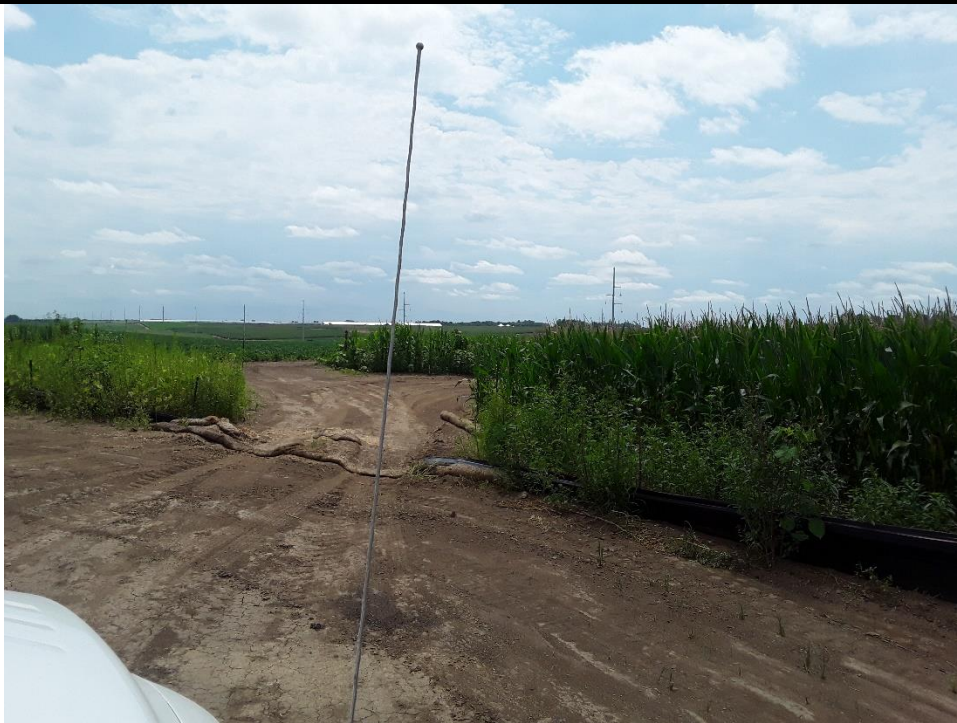
Substation, PP-3: Inefficient BMPs should be removed. Wattle being placed across road when not working to prevent sediment from leaving the substation area.
