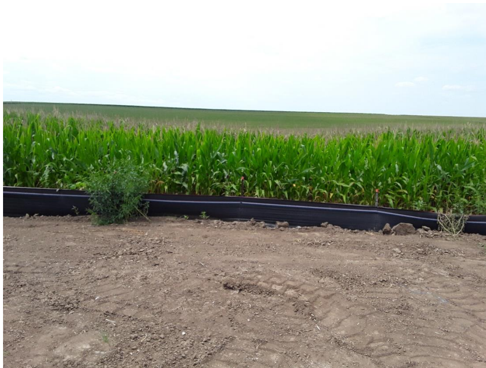
Substation, PP-2: Repaired silt fence on the west side of the substation. Silt fence is showing wear where attached to the supports. May need to be replaced if no longer efficient. Monitor in future inspections.
