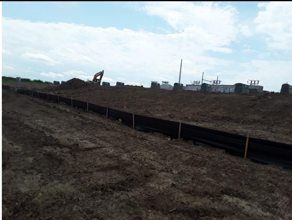
Substation, Photo Point (PP-1): Slopes on the east side of the substation have been disturbed after having been previously seeded for stabilization.
