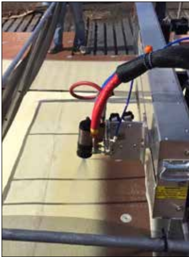
Our polyurethane spray foam robot is applying foam at an even 1.5" thickness across the roof which is 100% waterproof. This is creating a 100% seamless monolithic seal on the roof and an R-value of 20 with existing conditions.
