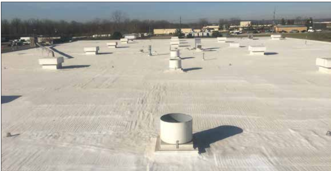
Granules are embedded in the top coat of silicone for toughness and durability.
