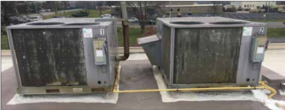
Walkpads applied around all serviceable mechanical units to provide non-slip conditions on a working or traffic surface.
