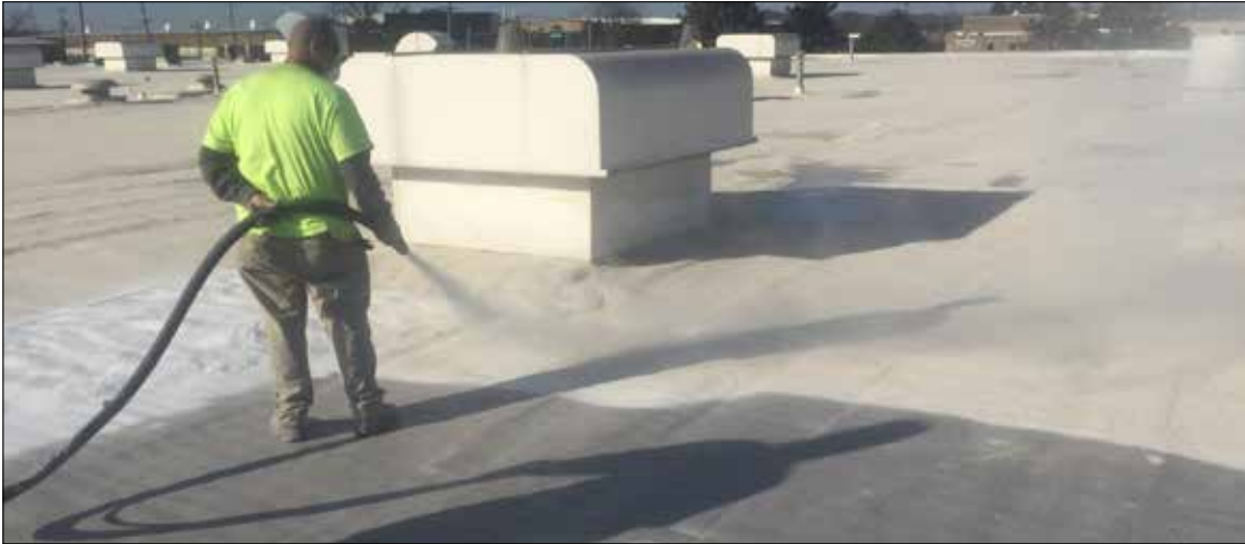
100,000 sq/ft of 1.5" with .5" insulation board spray foam roof and granule top coated silicone complete.
