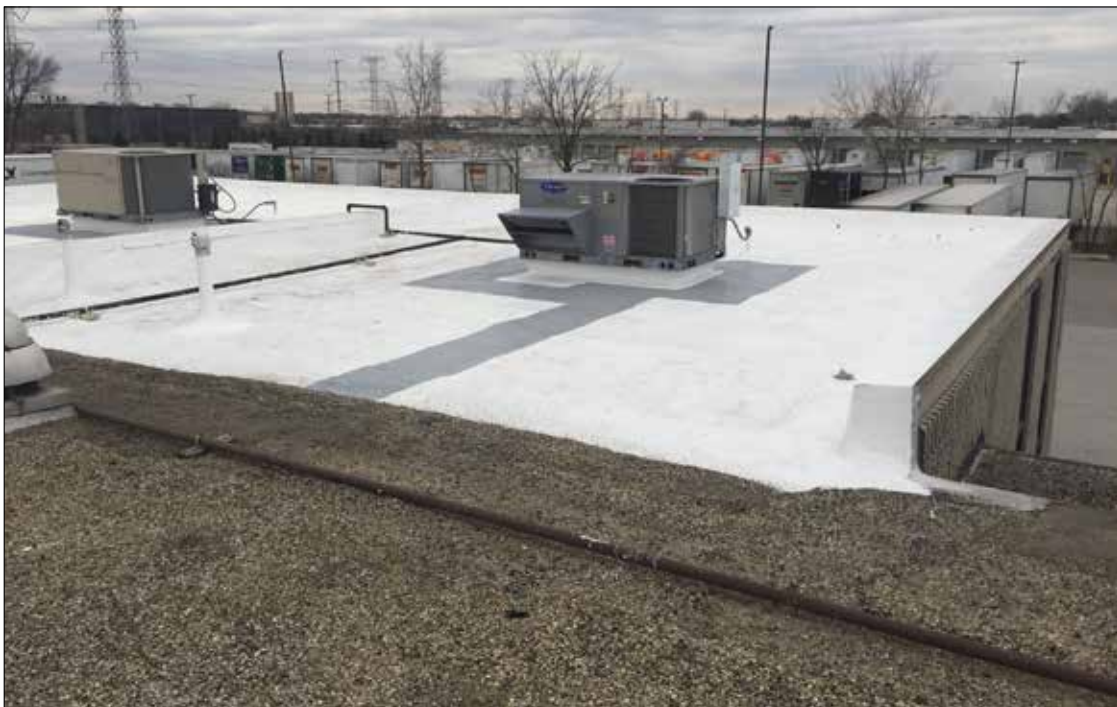
Finished silicone repair process on a gravel built-up roof.
