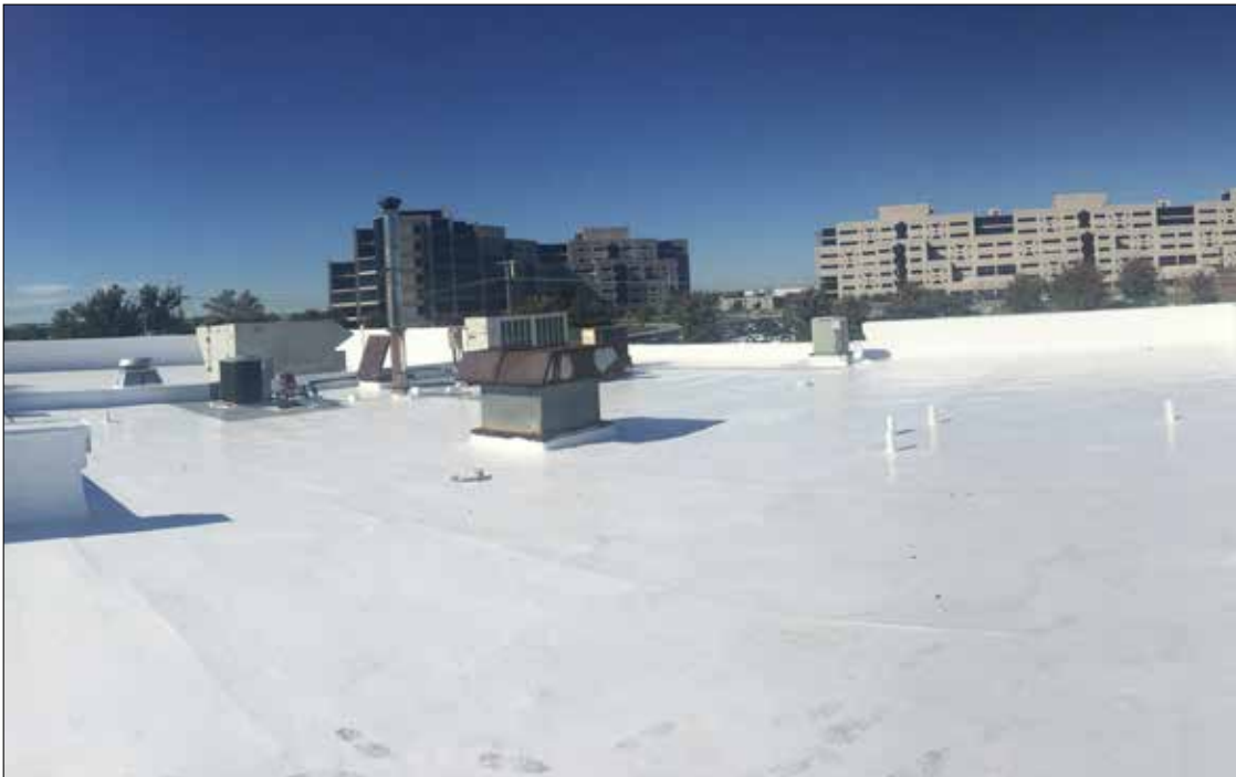
EPDM roof flashed and coated with high solids silicone at 2 gallons per 100 sq/ft for a 15-year manufacturer backed warranty.
