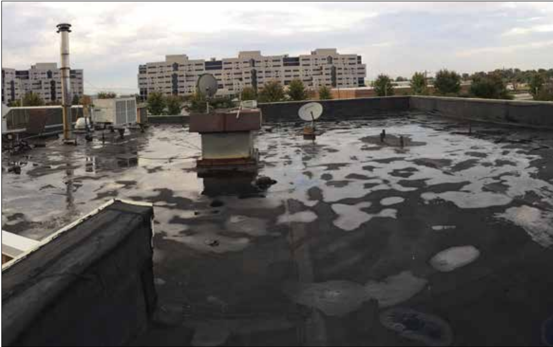
EPDM roof with failing seams and cracking membrane throughout the field. A perfect candidate for a restoration system.
