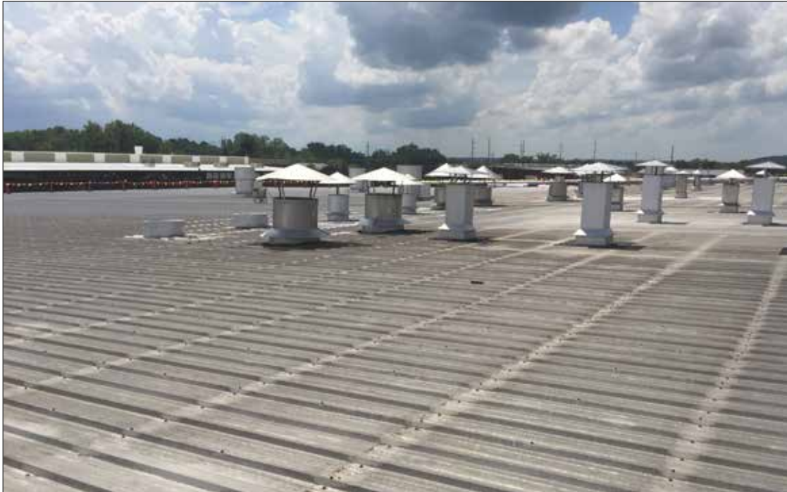
R-Panel Roof 180,000 sq ft. with engineered flashing, curbs, walk pads, crickets and expansion joints.
