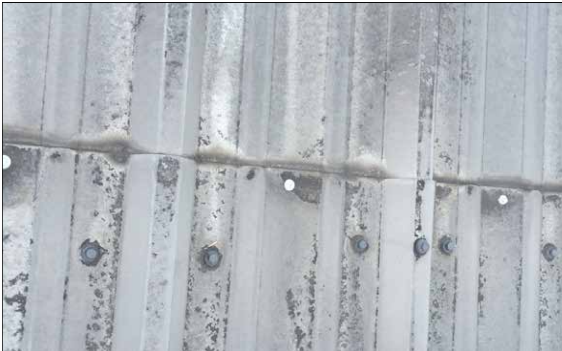
This picture shows a loose seam. We add 1-2 screws to each 12" length of seam as our engineering process requires.
