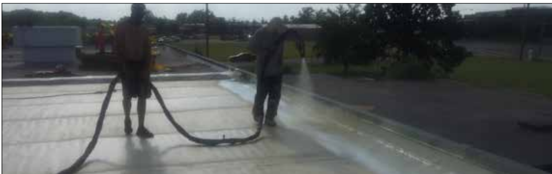
Custom cant strip created with spray foam at parapet walls to divert water to drains.
