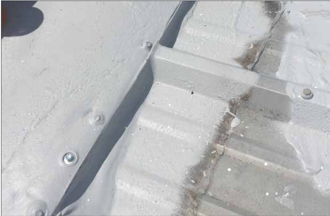
Shows a closer view of the screws added and the transition flashed with fiber flashant 40-50 mils thick.
