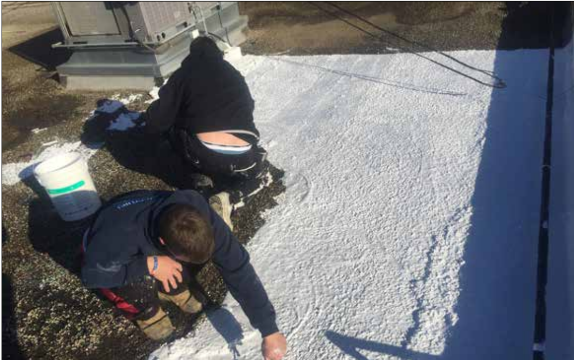
In process of repair. Coating with 40-70 mils of HS silicone.
