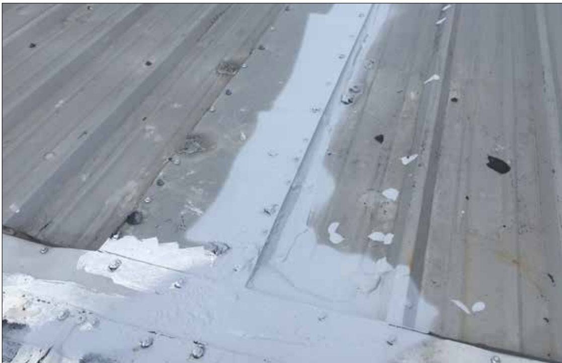
Shows a custom expansion joint bridge screwed down and sealed. Flashed with 40-50 mils of fiber flashant.
