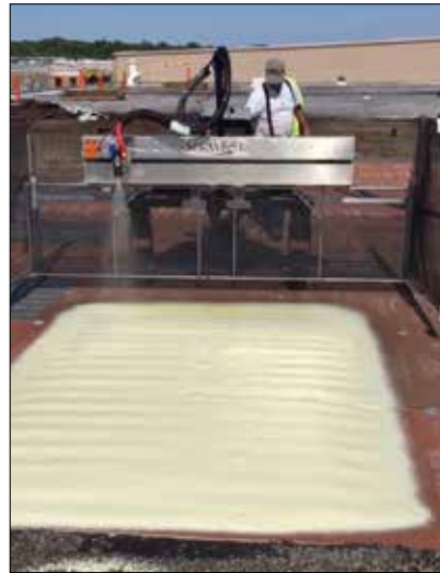
Our polyurethane spray foam robot is applying foam at an even 1.5" thickness across the roof which is 100% waterproof. This is creating a 100% seamless monolithic seal on the roof and an R-value of 20 with existing conditions.
