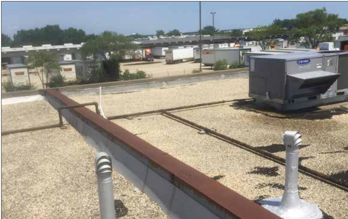
Before picture of a gravel topped built-up roof.
