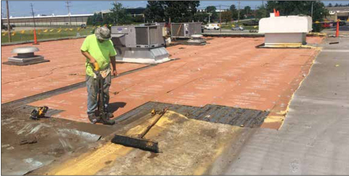
Plates and fasteners are being applied to fiber boards over top of the metal roof deck. Bad deck panels are replaced as needed.
