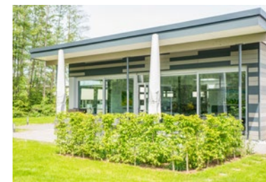
A place to meet and relax, just outside our canteen building
