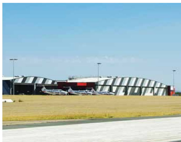
Police Airwing and Air Ambulance hangar facility
