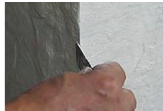
3. If there is a seam in the point, it needs to be repaired tightly with the same color caulking agent.
