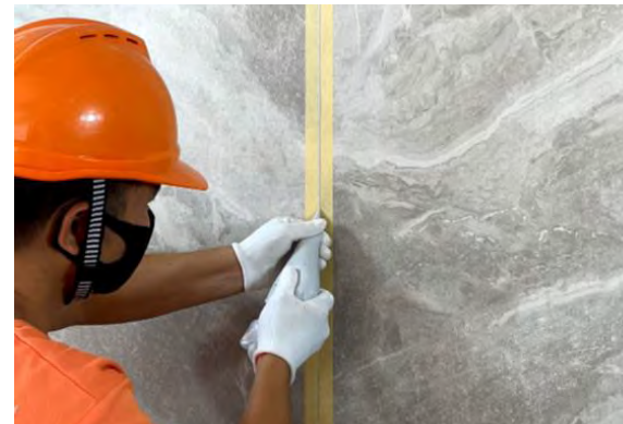
2. Caulk the seams with a triangular bag of caulk agent
