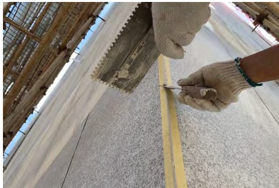
3. Wait for the caulk to semi-dry to clean the caulk agent out of the seam
