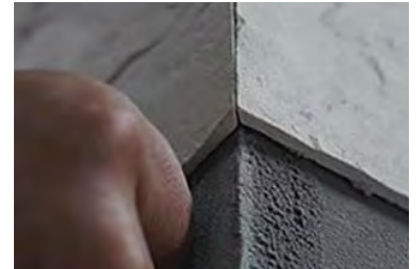
2. When sticking to the corner, the adhesive should be filled, and the two pieces of products should be compacted evenly by hand.
