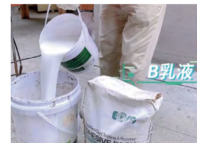
1.pour emulsion B into the barrel
