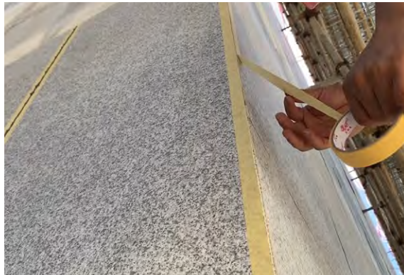
1. Paste masking paper along the external angle
