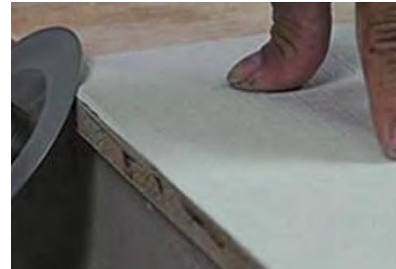
1. Grind a 45 bevel angle on the edge of the product with a small grinder (the smaller the bevel angle is during grinding, the easier it is to jump when pasting).
