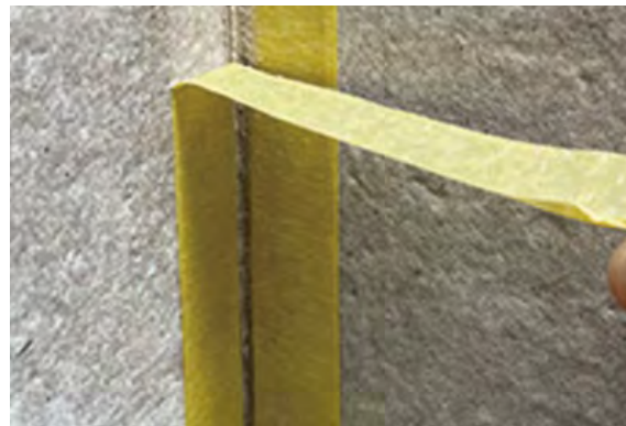
4. Tear off the masking paper, and in a semi-dry state, clean the overflow caulking agent with a sponge
