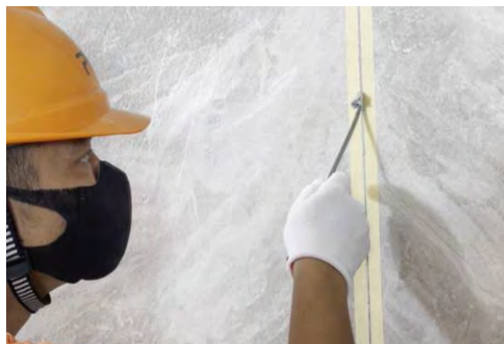
3. Clean the caulk agent out of the seams with a steel bar or trowel.
