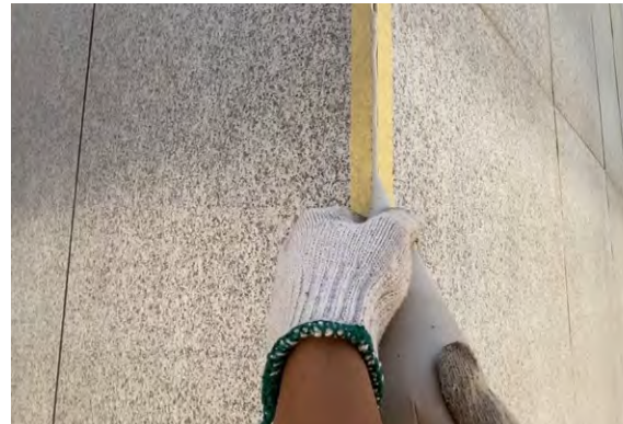
2. Caulk with a triangle bag of caulk
