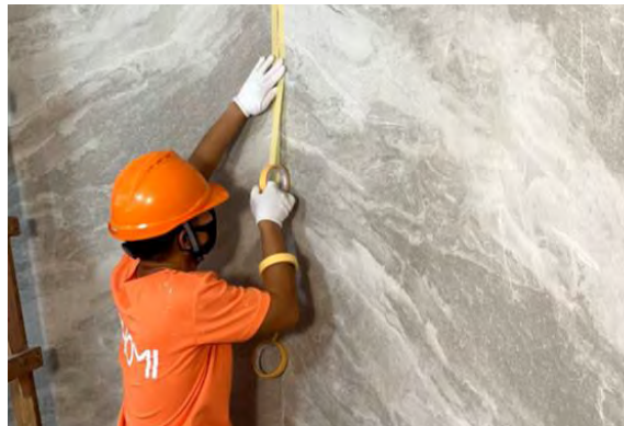
1. Paste the masking paper along both sides of the seams
