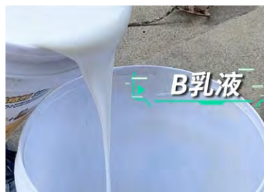
1.pour emulsion B into the barrel
