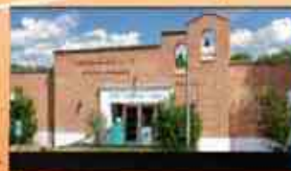
TUBAC COMMUNITY CENTER 50 BRIDGE RD.
