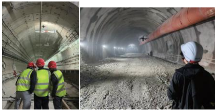
Tunnel Daily Inspection
