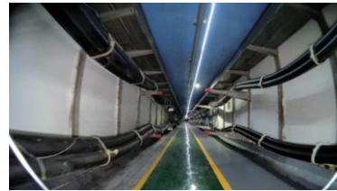
Common Utility Daily Inspection
