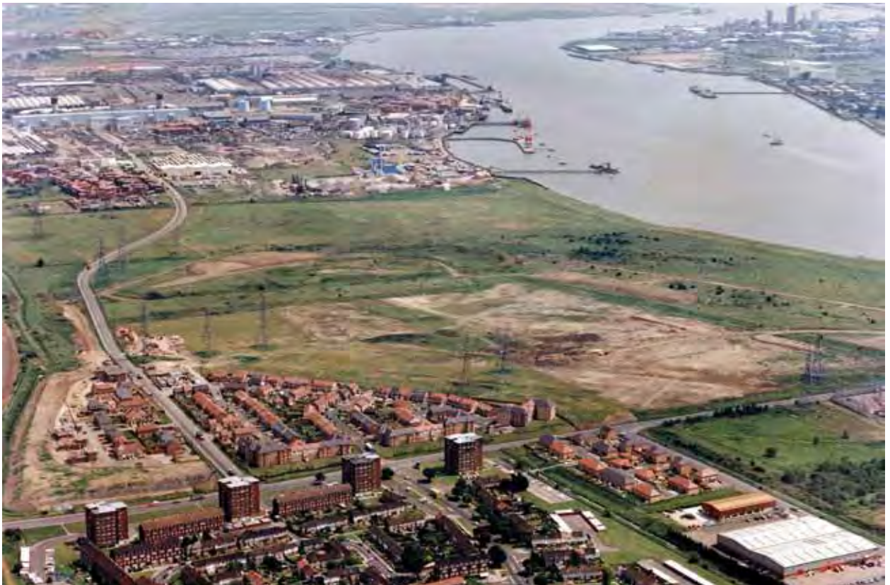
BARKING RIVERSIDE View to the East
