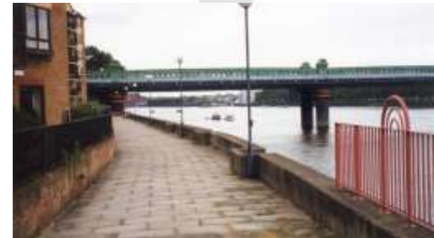
Fulham, above Putney Rail Bridge ~ Poor setting
