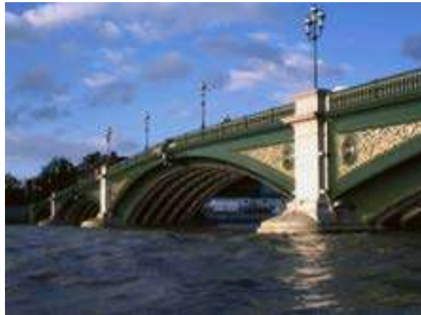
Battersea Bridge built by Sir Joseph Bazalgette in the late 1880's
