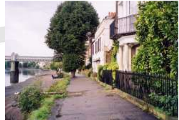
No.1 Strand on the Green and Kew Railway Bridge
