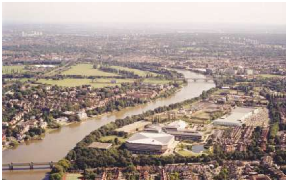
Aerial view of Character Reach No.1 Kew and Strand on the Green
