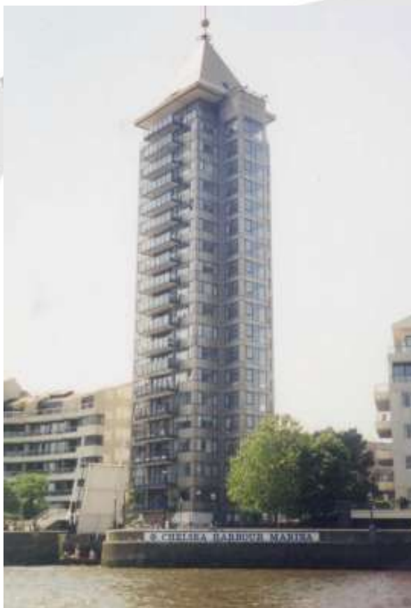
Belvedere Tower, Chelsea Tower
