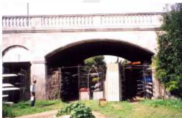
Potential to use arch under Chiswick Bridge for Thames Path
