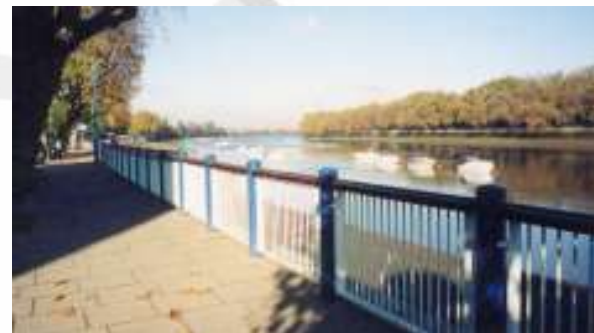
Balustrade Putney Embankment
