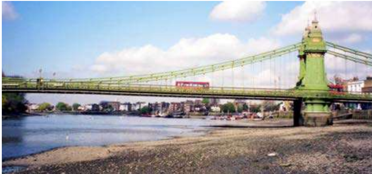
Hammersmith Bridge looking upstream
