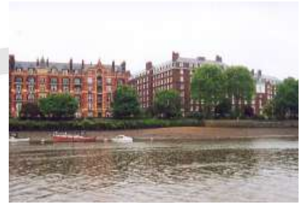
Mid-stream moorings off Ranelagh Gardens
