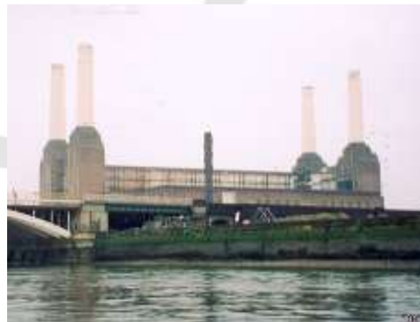
Battersea Power Station decommissioned
