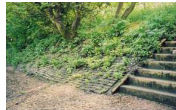
Sloping cobbled revetment
