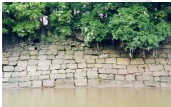
Sloping cobbled revetment, Duke's Meadow
