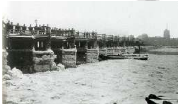
Old Fulham Bridge, 1881
