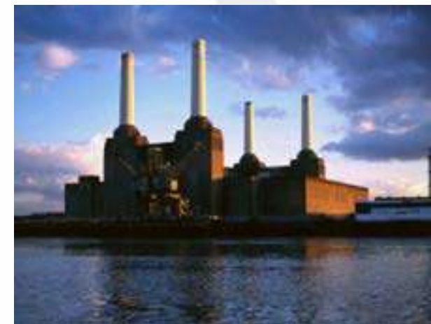
Sir Giles Gilbert Scott's Battersea Power Station
