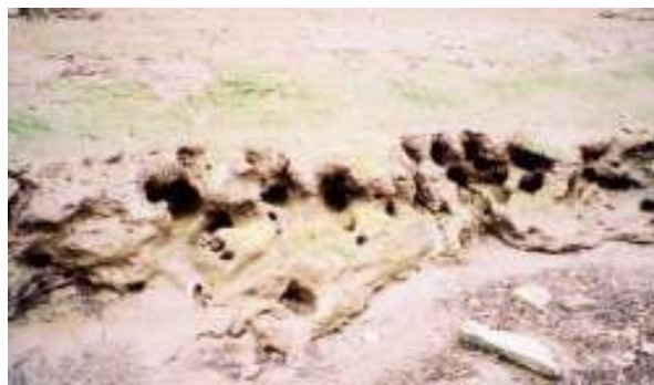
Damage caused by Mitten Crabs
