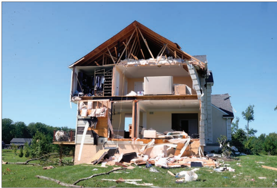
Homeowners clean up damage the day after a tornado touched down in Harrison Township, N.J., Sept. 2. The remnants of Hurricane Ida dumped historic rain over in the Northeast, with several deaths linked to flooding in the region as basement apartments suddenly filled with water and freeways and boulevards turned into rivers, submerging cars. Photo: Edward Lea /The Press of Atlantic City via AP
