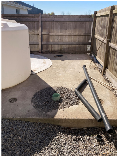
Photo 15 – Main Building Septic Holding Tank
