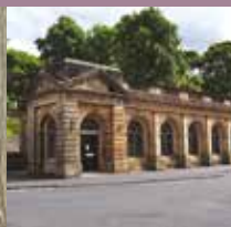
The Pump Room
