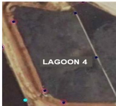
Figure 7.5. Arrangement of EBD MUD devices on Lagoon 4.
