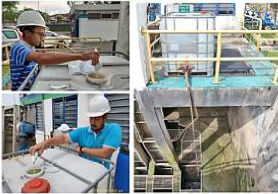
Fig. 3: Dosing of Bio-catalyst & EBD System installation at STP
