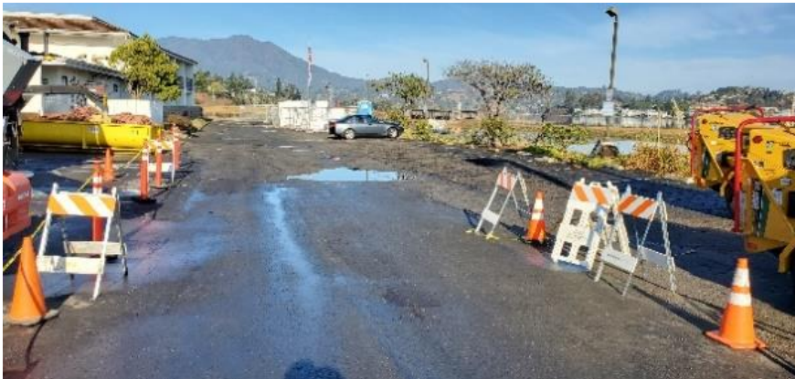
Beginning of Drainage Backflow
