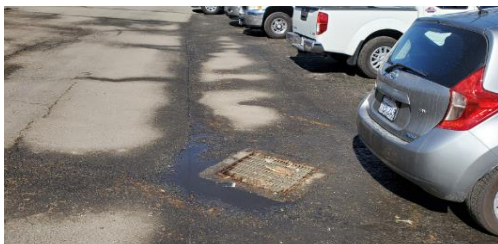
End of Drainage Backflow
