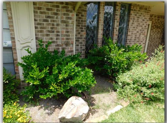
Inadequate clearance between the exterior wall cladding and grade (high soil or mulch) was observed. Inadequate clearance between the exterior wall cladding and grade should be corrected to prevent conducive conditions for wood destroying insects, water intrusion and deterioration of exterior siding materials.
