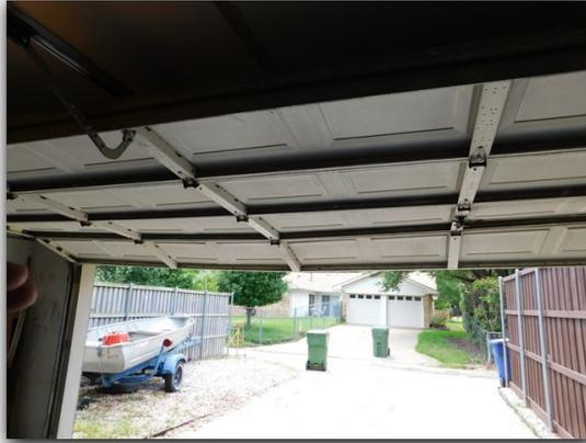
Damaged garage door weather stripping should be replaced.
