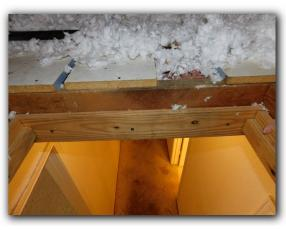
☑ Access doors from conditioned spaces to unconditioned spaces such as attics should be weather stripped and insulated to a level equivalent to the insulation on the surrounding surfaces. A wood framed or equivalent baffle or retainer should be installed when loose fill insulation is installed to assist in maintaining a consistent R-value.
