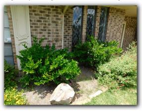
☑ Inadequate clearance between the exterior wall cladding and grade (high soil or mulch) was observed. Inadequate clearance between the exterior wall cladding and grade should be corrected to prevent conducive conditions for wood destroying insects, water intrusion and deterioration of exterior siding materials.
