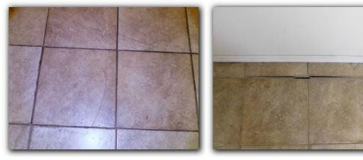
☑ Linear cracks in floor tiles were observed. Linear cracks in floor tiles may be an indication of movement, settlement, improper installation or other defects. The cause of linear cracks in floor tiles and grout should be further evaluated and repaired as needed.
