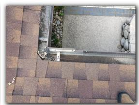
☑ All gutter downspouts should have downspout extensions or splash blocks installed to move run off water away from the foundation and to prevent erosion. Missing splash blocks and downspout extensions should be replaced.
