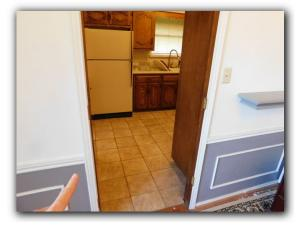
☑ Interior doors were observed to rub, stick or hit the door frames. Interior doors, that stick or hit the door frame may be an indication of movement, settlement or other defects. The cause of doors sticking or hitting door frames should be determined and repaired as needed.
