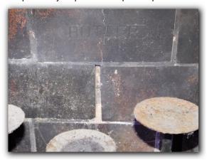
☑ The fireplace chimney lacks a metal cap and spark arrestor. This condition should be further evaluated and corrected as necessary. Masonry chimney caps are often not visible and are known to crack which allows moisture to penetrate the structure. Masonry chimney caps are considered inadequate by current building standards and should be replaced with metal caps.
