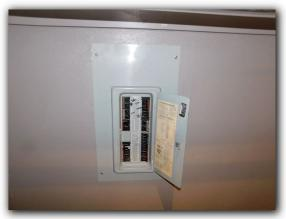
☑ The electrical panel was installed in a clothes closet. Under current electrical standards, this is not an accepted service panel location and is considered a SAFETY HAZARD. Electric service panels in clothes closets should be re-located to a safe and accessible location by a certified, licensed electrical specialist.
