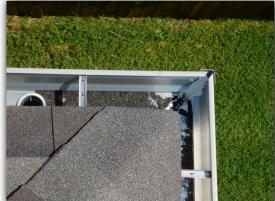
$\square$  The rain gutter downspout splash blocks were installed backwards. Splash blocks that are installed backwards do not perform as intended and may contribute to erosion.
