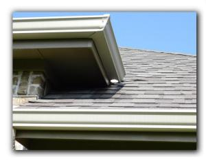
☑ Improperly sloped rain gutters were observed. Improperly sloped rain gutters create conducive conditions for siding deterioration, soffit/eave damage, water penetration and inadequate grade drainage.
