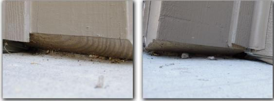
☑ Exterior sealants were deteriorated or missing in some areas. Sealants applied in appropriate locations prevents moisture intrusion and insect penetration.
