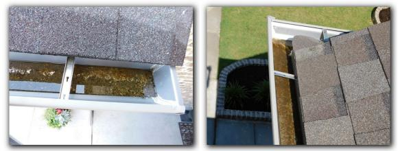
$\blacksquare$  The gutters and downspouts contained leaves and other debris and should be cleaned out to allow for proper drainage.
