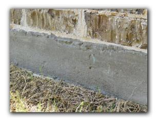
☑ Foundation perimeter beam corners have been sheared off (corner pop). This is a common condition in slab on grade foundations and should be repaired. Repairing corner pops is recommended to prevent moisture and wood destroying insect penetration.
