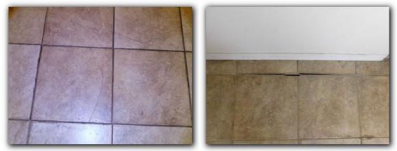
☑ Linear cracks in floor tiles were observed. Linear cracks in floor tiles may be an indication of movement, settlement, improper installation or other defects. The cause of linear cracks in floor tiles and grout should be further evaluated and repaired as needed.
