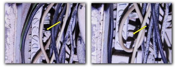
☑ Incorrect electrical conductor sizes were observed to be connected to breakers in the electric service panel. Incorrect electrical conductor sizes are a SAFETY HAZARD and create conducive conditions for overheating and or breaker tripping. Incorrect electrical conductor sizes should be further evaluated and repaired or replaced by a qualified electrical specialist.
