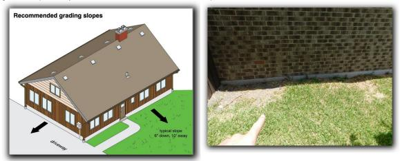
☑ High soil levels were observed at the foundation/brick line. 4 to 6 inches of the foundation perimeter beam should be visible. High soil levels may block weep holes and prevent proper wall ventilation. High soil levels create conducive conditions for wood destroying insects and water intrusion. High soil levels prevent the inspector from observing the foundation perimeter beam. Correction of inadequate grading clearance to exterior wall and foundation surfaces is recommended.
