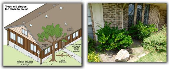
☑ Inadequate clearance between the exterior wall cladding and grade (high soil or mulch) was observed. Inadequate clearance between the exterior wall cladding and grade should be corrected to prevent conducive conditions for wood destroying insects, water intrusion and deterioration of exterior siding materials.
