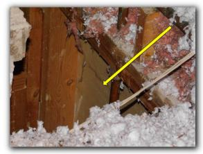
$\square$  The lack of roof decking expansion clips was observed. The lack of roof decking expansion clips may be an indication of improperly installed roof decking.
