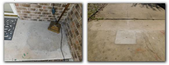
☑ A cosmetic skim coat of mortar material has been installed over the exterior foundation perimeter beam that may conceal defects that would otherwise be observed. Foundation skim coats also create conducive conditions for wood destroying insects.
