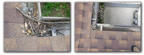
All gutter downspouts should have downspout extensions or splash blocks installed to move run off water away from the foundation and to prevent erosion. Missing splash blocks and downspout extensions should be replaced.
