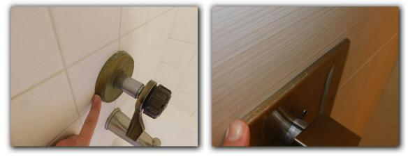
$\square$  The tub/shower tile grout and sealants were observed to be in need of repair or replacement to prevent water penetration at interior walls. When tub/shower tile grout and sealants are damaged, there may be concealed water damage and or wood destroying insect damage.
