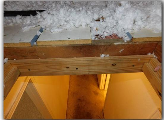
☑ Access doors from conditioned spaces to unconditioned spaces such as attics should be weather stripped and insulated to a level equivalent to the insulation on the surrounding surfaces. A wood framed or equivalent baffle or retainer should be installed when loose fill insulation is installed to assist in maintaining a consistent R-value.
