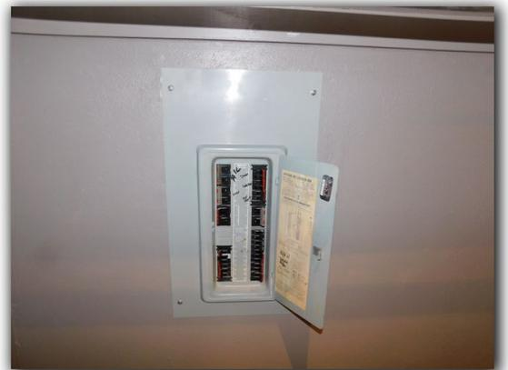
The electrical panel was installed in a clothes closet. Under current electrical standards, this is not an accepted service panel location and is considered a SAFETY HAZARD. Electric service panels in clothes closets should be re-located to a safe and accessible location by a certified, licensed electrical specialist.
