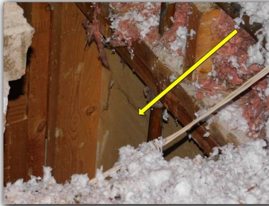
The lack of roof decking expansion clips was observed. The lack of roof decking expansion clips may be an indication of improperly installed roof decking.
