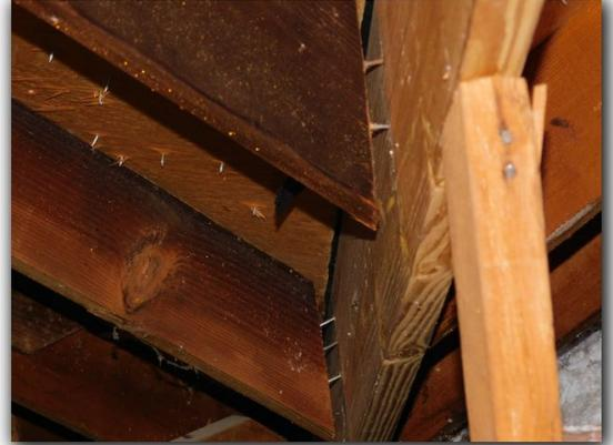
Soffit vents were observed to be dirty, blocked by insulation or debris. Clogged soffit vents are an indication of inadequate attic ventilation and should be repaired as needed.
