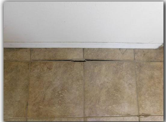
Linear cracks in floor tiles were observed. Linear cracks in floor tiles may be an indication of movement, settlement, improper installation or other defects. The cause of linear cracks in floor tiles and grout should be further evaluated and repaired as needed.
