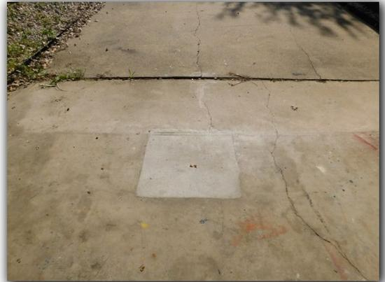
A cosmetic skim coat of mortar material has been installed over the exterior foundation perimeter beam that may conceal defects that would otherwise be observed. Foundation skim coats also create conducive conditions for wood destroying insects.
