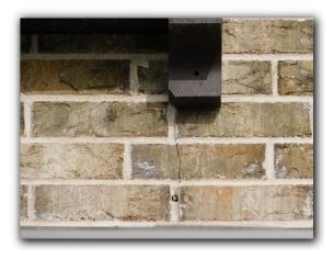
☑ Areas of the exterior brick veneer siding overhang the foundation and appeared to be improperly installed. Brick veneer siding that does not rest on the foundation may not be properly supported.
