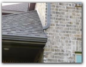
☑ All gutter downspouts should have downspout extensions or splash blocks installed to move run off water away from the foundation and to prevent erosion. Missing splash blocks and downspout extensions should be replaced.
