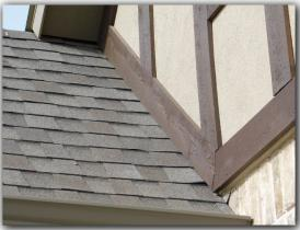
☑ Roof covering flashings were observed to be lifting, damaged or improperly installed and were in need of repair or replacement. Lifting, damaged or improperly installed flashings may allow water penetration.
