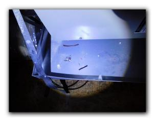
☑ The cooling equipment condensation overflow pan or drain lines installed above ceilings were not equipped with water or moisture sensors/alarms. Cooling equipment condensation drain pans or drain line sensors and alarms should be installed at cooling equipment installed above ceilings for additional protection against water damage.
