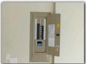
☑ The electric service panel breaker use was not correctly labeled. Each electric service panel breaker should be adequately labeled as to what appliance or circuit it serves.
