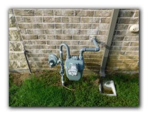
☑ There were gas fired appliances that did not have a "drip leg" installed. Under current construction standards, drip legs are required at the black iron gas pipe prior to a flexible gas line connection.
