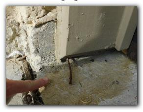
☑ Exterior sealants (caulking) were deteriorated or missing in some areas. Sealants applied in appropriate locations prevents moisture intrusion and insect penetration.
