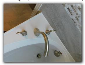
☑ The tub/shower water supply fixtures lacked adequate sealant at the wall. Tub/shower water supply fixtures should be properly sealed at the wall to prevent water damage.
