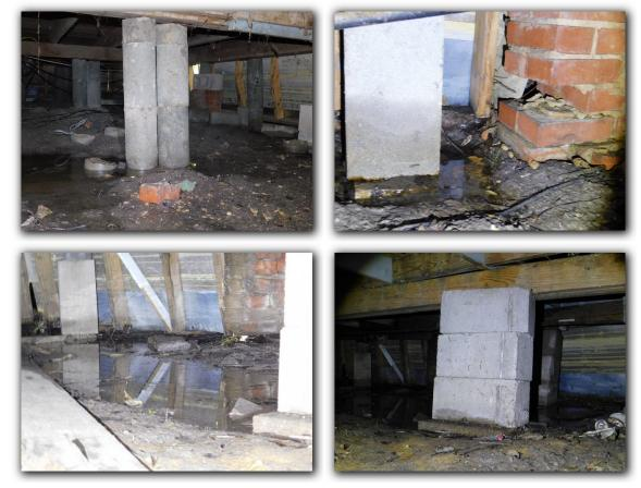
$\square$  No subfloor insulation was installed in the crawl space between the floor joists. Subfloor insulation prevents moisture intrusion and energy loss through the living space flooring.
