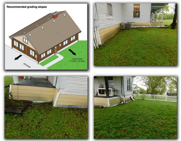
☑ Ponding next to the foundation was observed. Any area where the ground or grade does not slope away from the structure is to be considered an area of improper drainage. Corrective measures may be needed if the water stands within 10-feet of the foundation perimeter beam for more than 24-hours. Grading improvements are needed to direct run off water away from the structure. Recommended slope away from the foundation is 6 inches per 10 feet.
