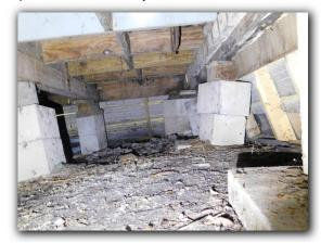
☑ Crawl space vents should be installed within three feet of building corners. The crawl space ventilation was inadequate. Inadequate crawl space ventilation creates conducive conditions for structural damage, wood rot, moisture damage and wood destroying insects.
