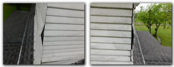
☑ The exterior wood trim was observed to have some deterioration and/or damage. Damaged and deteriorated exterior wood trim should be repaired to prevent wall damage, moisture penetration and wood destroying insects.
