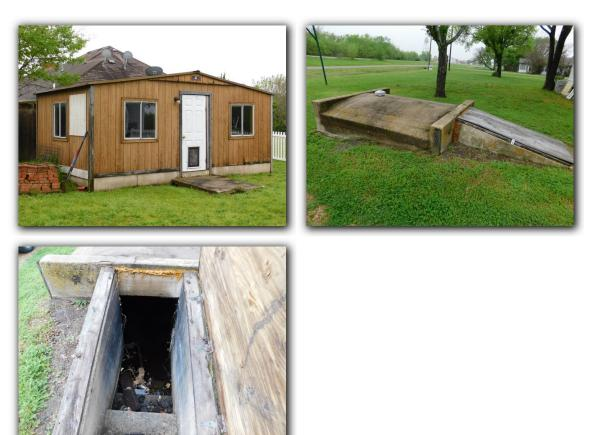
☑ The exterior outbuilding wood veneer siding was observed to have some deterioration and/or damage. Damaged and deteriorated outbuilding exterior wooden siding should be repaired to prevent wall damage, moisture penetration and wood destroying insects.
