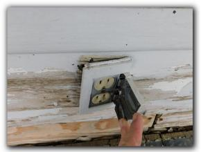
☑ Painted electrical receptacles were observed. Painted electrical receptacles are considered damaged and should be replaced by a certified, licensed electrical specialist for improved safety and performance.
