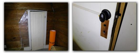
☑ Interior doors which drift closed were observed. Interior doors, which drift, are an indication of movement, settlement or other defects. The cause of door drift should be determined and repaired as needed.
