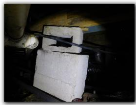
☑ Leaning piers were observed in the crawl space. Leaning piers may not provide adequate support for the structure. The inspector recommends that the foundation be further evaluated and repaired as needed by a certified, licensed foundation specialist.
