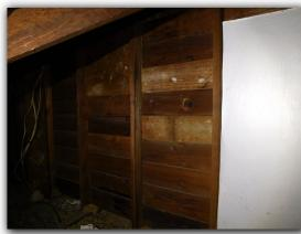
☑ Loose and or damaged insulation was observed in the attic space. Loose or damaged insulation may allow greater than normal loss of conditioned air and should be repaired.
