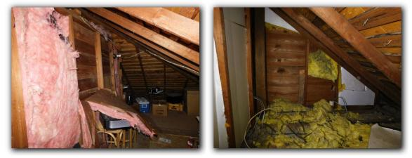
$\square$  The attic insulation depth or thickness was inadequate. The recommended depth of attic floor insulation is 13+ inches to achieve an R38 rating. Inadequate attic insulation depth or thickness may allow greater than normal loss of conditioned air.
