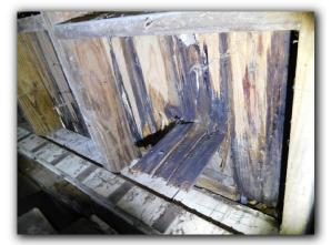
☑ Deteriorated pier and beam conditions were observed. Deterioration of pier and beam supports should be repaired to prevent adverse effects to the foundation and structure. Deteriorated pier and beam components should be repaired or replaced by a certified, licensed foundation specialist.
