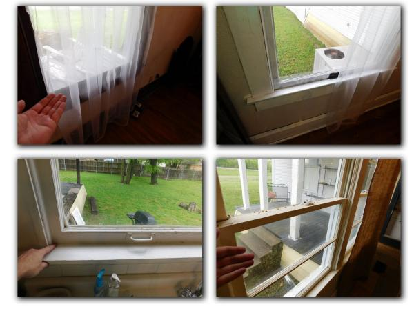
☑ One or more of the bedroom windows have been painted shut. At least one window in each bedroom should open fully, with free access to the outdoors. Lack of an operable window in each bedroom is a FIRE SAFETY HAZARD and should be repaired prior to being occupied.
