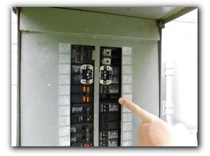
☑ Unused knockouts in the electric service panel were observed to be missing knockout covers (where conductors may pass through electrical cabinet walls). Missing knockout covers or unused conductor openings should be covered with electrical knockout covers to prevent the unwanted entry of pests, moisture or other items. Lack of an electrical knockout cover at unused conductor openings is considered a SAFETY HAZARD and should be repaired as needed by a qualified electrical specialist.
