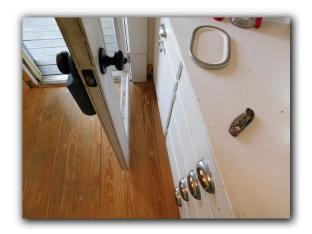
☑ Damaged or missing exterior door weather stripping should be replaced. Missing or damage exterior door weather stripping creates conducive conditions for moisture intrusion and conditioned air loss.
