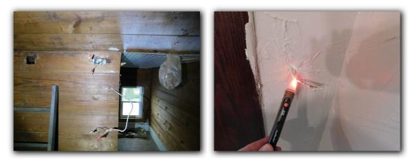
☑ Electrical junction / receptacle boxes were observed to be missing covers. All electrical conductor connections should be installed in sealed junction boxes for reasons of safety. Improperly terminated electrical conductors should be repaired by a certified, licensed electrical specialist.
