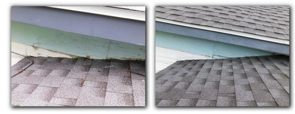
☑ Exposed or lifting fasteners or nail heads were observed at the roof coverings. Exposed or lifting fasteners or nail heads may allow water penetration and were in need of repair.
