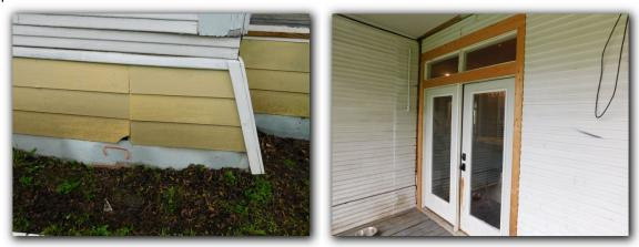
☑ The exterior wood veneer siding was observed to have some deterioration and/or damage. Damaged and deteriorated exterior wooden siding should be repaired to prevent wall damage, moisture penetration and wood destroying insects.
