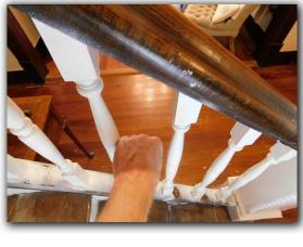
☑ Inadequate stairway headroom was observed. Under current building standards the minimum headroom in all parts of the stairway shall not be less than 6 feet 8 inches measured vertically from the slope of the plane adjoining the tread nosing or from the floor surface of the landing or platform.
