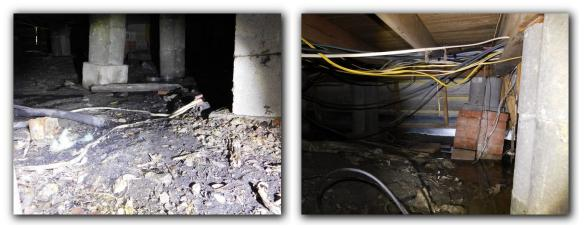
☑ Knob and tube electrical components were observed. Knob and tube type electrical systems are no longer an accepted electrical standard. Knob and tube electrical systems are considered a SAFETY HAZARD under current building standards. Knob and tube electrical systems should be further evaluated and replaced as needed by a certified, licensed electrical specialist.
