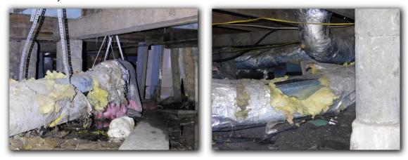
☑ Ductwork installed in the crawl space was observed to be in contact with the ground and should be properly supported.
