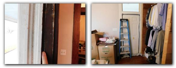
$\blacksquare$  Safety glass was not installed in exterior doors side lights. Lack of exterior door side light safety glass is a SAFETY HAZARD.
