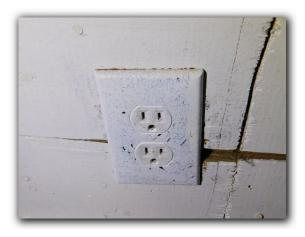
☑ Electrical receptacles, switches and or covers were observed to be loose, damaged, missing or missing screws and were in need of repair. Damaged or missing electrical receptacles or switches should be repaired by a certified, licensed electrical specialist.
