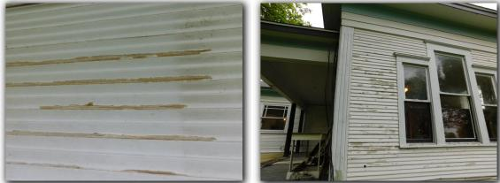
☑ Peeling, damaged or deteriorating paint, stain and/or sealant was observed at the exterior trim. Peeling, damaged and deteriorating paint or sealant should be repaired to prevent moisture penetration and deterioration of materials.
