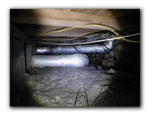
☑ The absence of airflow at heating/cooling supply registers was an indication of disconnected or damaged ducts. The cause of inadequate airflow at the heating/cooling supply registers should be determined and repaired as needed.
