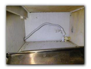
☑ Older style gas valves require a tool to operate. Under current building standards, gas valves should be operable by hand for reasons of safety.
