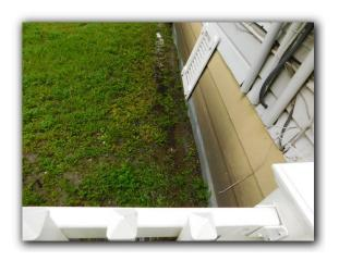
☑ The structure has been built below the public street grade. Extra caution should be taken to prevent any possible water intrusion to the structure. Do not build flowerbeds that will cause a damming effect and hold water next to the structure. Positive drainage should always be maintained.
