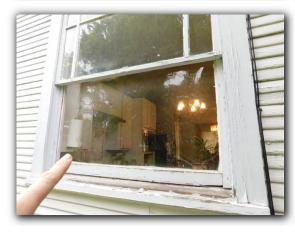
☑ The window above the tub/shower did not appear to have a safety glass etching or label. Glass less than 5' above the tub/shower should be tempered safety glass. Lack of safety glass in required locations is a SAFETY HAZARD and should be replaced.
