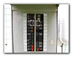
☑ The electric service panel electrical conductors have not been properly secured or protected from the sharp edges and or the dead front cover of the cabinet. Electrical conductors that are in contact with the service panel dead front cover and not protected from sharp edges are a SAFETY HAZARD and should be repaired by a qualified electrical specialist.
