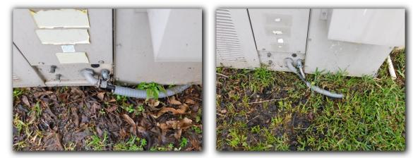
☑ Improperly terminated electrical conductors were observed. All electrical conductor connections should be installed in sealed junction boxes for reasons of safety. Improperly terminated electrical conductors should be repaired by a certified, licensed electrical specialist.
