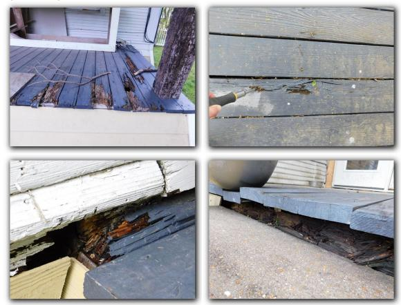
$\boxtimes$  Wooden deck construction materials were observed to be in contact with the ground. Wood to ground contact at decking construction materials creates conducive conditions for wood rot and wood destroying insects.
