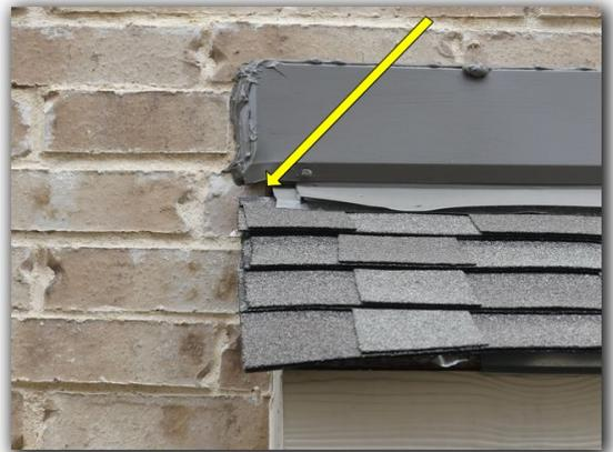
Current construction standards require a kick out flashing at the roof coverings and wall intersections. Kick out flashings prevent water leaks, damage and discoloration to walls.
