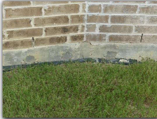
Cracks and damage were observed in the cosmetic skim coat covering the foundation slab. Cracks in the cosmetic skim coat should be repaired. Moisture penetration may allow further deterioration of the cosmetic skim coat.
