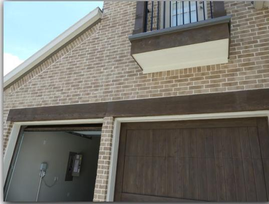
Weep holes were not installed in the brick/stone masonry above the windows in required locations. Under current building standards, weep holes should be installed in the brick/stone masonry above windows to provide proper wall ventilation.
