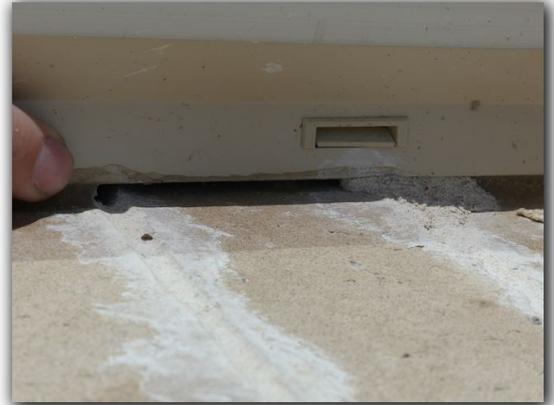
The window frames were observed to be damaged. Damaged windows may allow moisture penetration, conditioned air loss and insect penetration and should be repaired.
