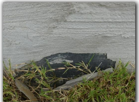
Foundation slab corners have been sheared off (corner pop). This is a common condition in slab on grade foundations and should be repaired. Repairing corner pops is recommended to prevent moisture and wood destroying insect penetration.
