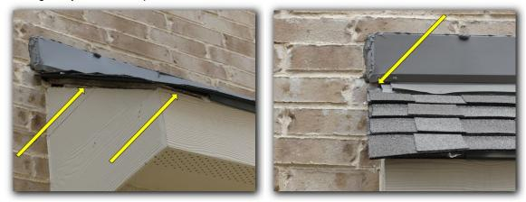
☑ Current construction standards require a kick out flashing at the roof coverings and wall intersections. Kick out flashings prevent water leaks, damage and discoloration to walls.
