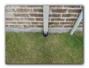
☑ The secondary roof rain gutter lacks a downspout. Lack of a downspout at secondary roof rain gutters may allow localized deterioration and premature wear of the roof covering materials.
