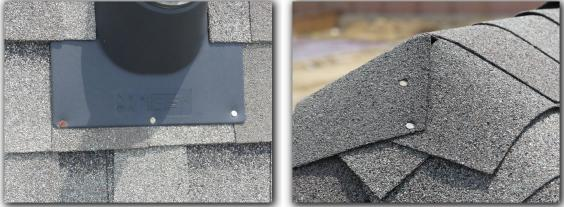
☑ Roof covering drip edge and flashings were observed to be missing, damaged or improperly installed and were in need of repair or replacement. Missing, damaged or improperly installed flashings may allow water penetration.
