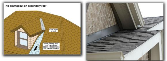
☑ Damaged or improperly installed rain gutters and downspouts should be repaired. Damaged or leaking rain gutters and downspouts create conducive conditions for siding deterioration, soffit/eave damage, roof covering damage, water penetration and inadequate grade drainage.
