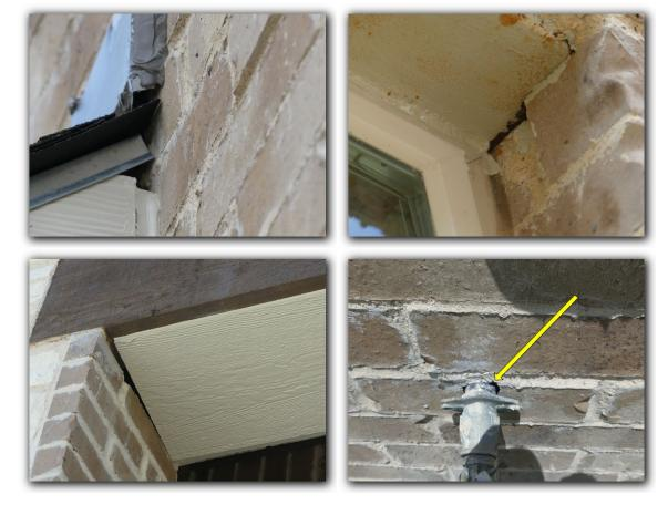
☑ Weep holes were not installed in the brick/stone masonry above the exterior doors in required locations. Under current building standards, weep holes should be installed in the brick/stone masonry above exterior doors to provide proper wall ventilation.
