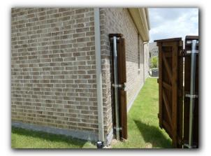
☑ Exterior sealants (caulking) were deteriorated or missing in some areas. Sealants applied in appropriate locations prevents moisture intrusion and insect penetration.
