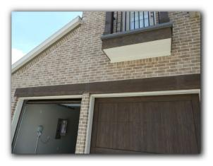
☑ Weep holes were not installed in the brick/stone masonry above the windows in required locations. Under current building standards, weep holes should be installed in the brick/stone masonry above windows to provide proper wall ventilation.
