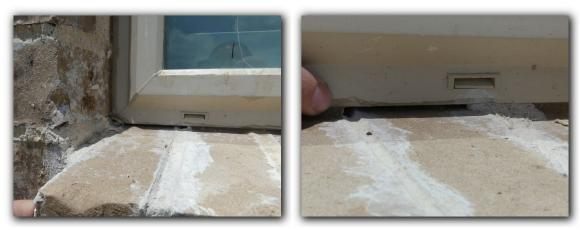
☑ The window frames were observed to be damaged. Damaged windows may allow moisture penetration, conditioned air loss and insect penetration and should be repaired.
