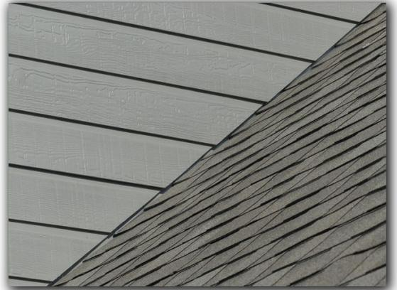
Roof covering flashings were observed to be lifting and were in need of repair. Lifting, damaged or improperly installed flashings may allow water penetration.
