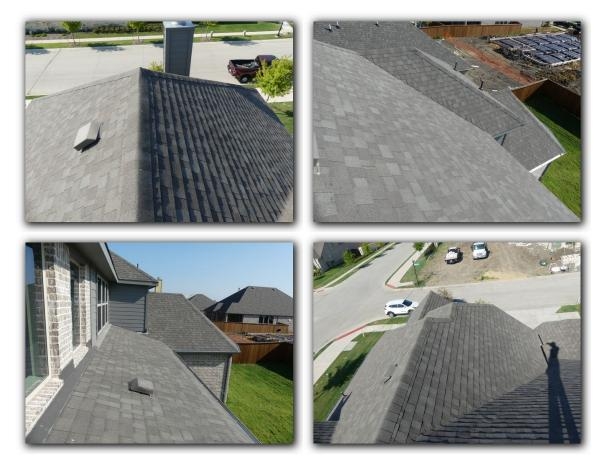
☑ There were indications of impact damage on the roof covering. Impact damaged roof covering shingles may allow further deterioration of the roof covering, deterioration of the roof structure,
