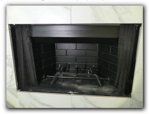
☑ The fireplace firebox was not sealed at the hearth or lintel and was a SAFETY HAZARD. Inadequate fireplace seals may allow heat to transfer to flammable materials and is a SAFETY HAZARD that should be repaired by a qualified fireplace specialist.
