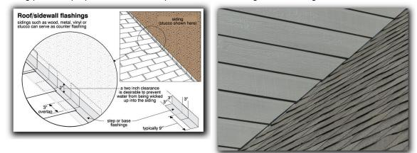
☑ Roof covering flashings were observed to be lifting and were in need of repair. Lifting, damaged or improperly installed flashings may allow water penetration.
