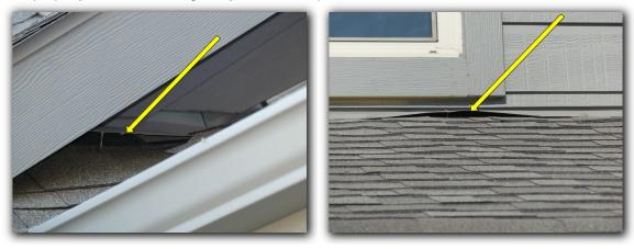
I Current construction standards require a kick out flashing at the roof coverings and wall
