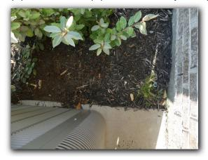
☑ The heavy foliage at and around the outside condenser/coils should be trimmed back a minimum of 18-inches for proper air circulation. Lack of adequate air flow at the exterior HVAC equipment may result in equipment damage, inadequate performance, reduced equipment life or other defects.
