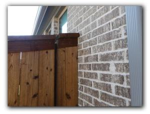
☑ One or more cracks were observed at the exterior brick/stone veneer masonry walls. Cracks in exterior brick/stone veneer wall cladding are indications that some movement or settlement has occurred. The inspector recommends that cracks in exterior walls be repaired and closely monitored. If concerns about the current or future foundation performance exist, the inspector recommends further evaluation by a certified, licensed foundation specialist.
