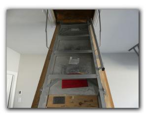
☑ The attic access stair in the vehicle storage area (garage) weatherstripping was missing or damaged andr was not fire rated and may allow vehicle storage area vapors to penetrate the attic and/or living area (SAFETY HAZARD).
