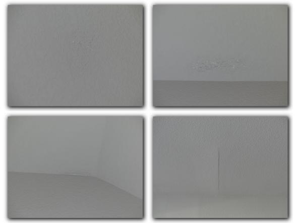
☑ Several interior ceiling cracks were observed which is an indication of structural settling, movement or other defects. Ceiling drywall, texture and paint cracks should be repaired and monitored over time for additional movement.
