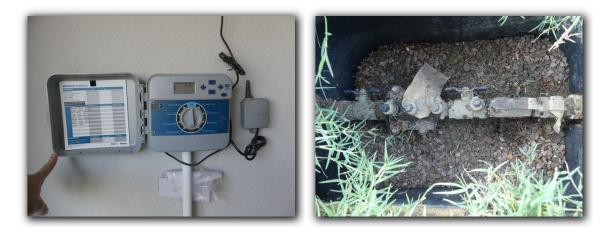
☑ The landscape irrigation system electrical grounding wire were loose and should be repaired.
