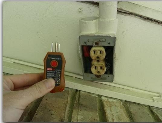
Current building standards require a GFCI protected electrical receptacle near the exterior HVAC equipment for technician use.
