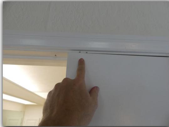
Interior doors which drift closed were observed. Interior doors, which drift, are an indication of movement, settlement or other defects. The cause of door drift should be determined and repaired as needed.
