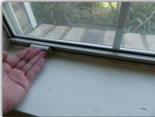
Damaged window lift supports were observed. Damaged window lift supports may not hold windows in the open position and may allow glass or window frame damage. Damaged window lift
