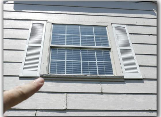
Windows were observed to be missing cap flashing. Missing window flashing should be repaired or replaced as needed.
