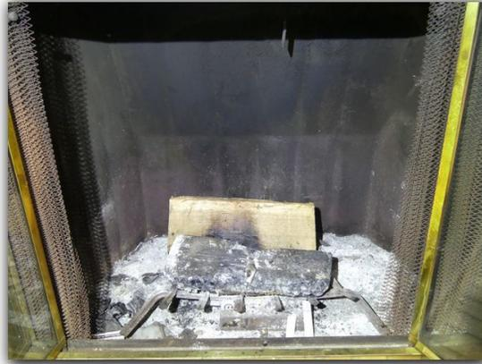
The fireplace and chimney flue needs to be cleaned by a qualified chimney sweep. A creosote or soot build-up was observed in the visible areas and was a SAFETY HAZARD at the time of the inspection. A creosote or soot build-up may be flammable and should be corrected prior to fireplace use.
