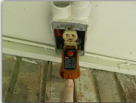
One or more 220V electrical receptacle was observed to be without electric power. The reason for a lack of electric power at 220V electrical receptacles should be determined and repaired as needed by a certified, licensed electrical specialist.
