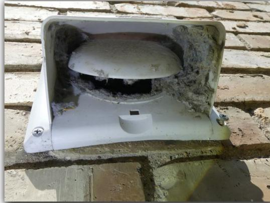
The dryer vent flapper was stuck in open position and was in need of repair or replacement. Dryer vent flappers that are stuck in the open position may allow moisture, insect and unwanted wildlife intrusion.
