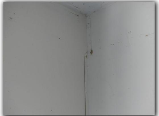
Interior drywall corner tape was observed to be pulling and twisting where walls and or ceilings intersect. This condition is related to adverse foundation or structural performance and should be further evaluated by a foundation or structural specialist and repaired as necessary.
