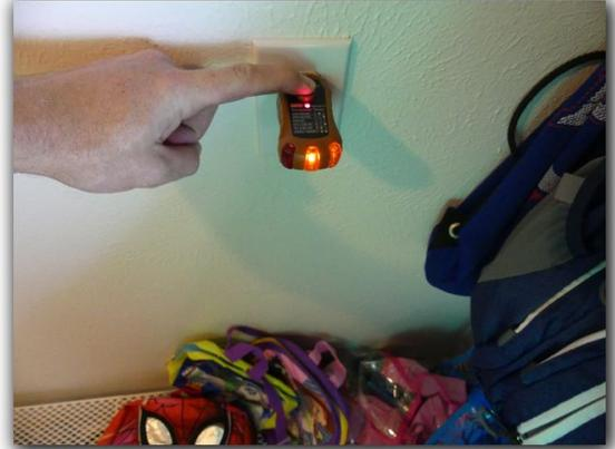
Garage electrical receptacles that are not connected to a ground fault circuit interrupter (GFCI) device are a SAFETY HAZARD. Under current electrical standards, all of the garage receptacles should have GFCI protection.
