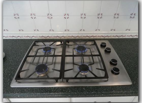
Missing and or damaged control knob indicators on the range/cooktop/oven should be repaired or replaced.
