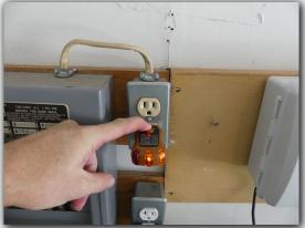
☑ Exterior electrical receptacles were observed to lack ground fault circuit interrupter (GFCI) device protection. Under current electrical standards, all of the exterior receptacles should have GFCI protection. Lack of GFCI protection in required locations is a SAFETY HAZARD.
