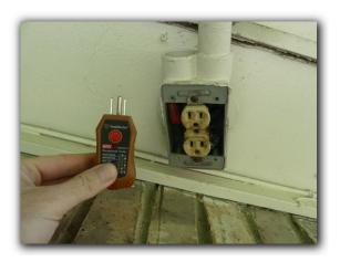
☑ Current building standards require a GFCI protected electrical receptacle near the exterior HVAC equipment for technician use.
