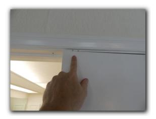
☑ Interior doors which drift closed were observed. Interior doors, which drift, are an indication of movement, settlement or other defects. The cause of door drift should be determined and repaired as needed.
