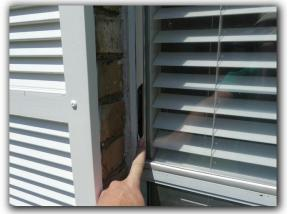
☑ Windows that are difficult to open or close were observed. The cause of windows that are difficult to open or close should be determined and repaired as needed.
