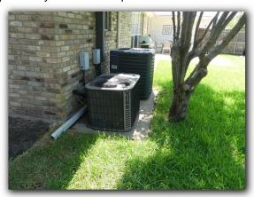
☑ The exterior HVAC equipment was not installed 3" above grade and was in need of repair. Inadequate elevation of the exterior HVAC equipment may allow moisture to penetrate the equipment, reduce equipment life and may affect performance.
