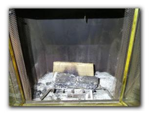
☑ The fireplace and chimney flue needs to be cleaned by a qualified chimney sweep. A creosote or soot build-up was observed in the visible areas and was a SAFETY HAZARD at the time of the inspection. A creosote or soot build-up may be flammable and should be corrected prior to fireplace use.
