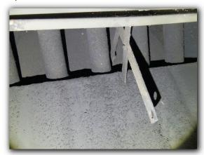
☑ The fireplace firebox brick/mortar was not sealed at the hearth or lintel and was a SAFETY HAZARD. Inadequate fireplace seals may allow heat to transfer to flammable materials and is a SAFETY HAZARD that should be repaired by a qualified fireplace specialist.
