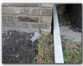
☑ Tree(s) in close proximity to the foundation were observed. The buyer should consider removal of the tree(s) or the installation of a root barrier to reduce the possibility of damage to the foundation from tree roots and moisture removal.
