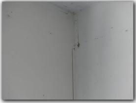
☑ Interior drywall corner tape was observed to be pulling and twisting where walls and or ceilings intersect. This condition is related to adverse foundation or structural performance and should be further evaluated by a foundation or structural specialist and repaired as necessary.
