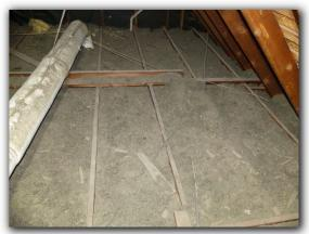
☑ The soffit vents lack baffles in the attic to prevent insulation or other materials from blocking the soffit vents.
