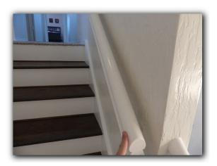
☑ The stairway handrail height was observed to be inadequate and was a SAFETY HAZARD. Under current building standards, the stairway handrail height should be 34"-36" and should be corrected prior to closing.
