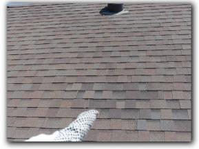
☑ Composition shingle tab granules were observed to be thinning on the roof covering. You are encouraged to have your insurance company and a certified, licensed roofing contractor physically inspect the roof, prior to closing, to fully evaluate the insurability and condition of the roofing material.
