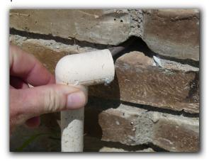
$\ensuremath{\square}$  The landscape irrigation system had missing and/or damaged sprinkler heads that should be replaced.
