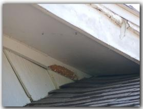
☑ Damaged or missing attic gable vents or vent screens should be repaired to prevent wildlife penetration and other defects.
