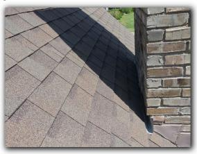
☑ The fireplace chimney lacks a metal cap. This condition should be further evaluated and corrected as necessary. Masonry chimney caps are often not visible and are known to crack which allows moisture to penetrate the structure. Masonry chimney caps are considered inadequate by current building standards and should be replaced with metal caps.
