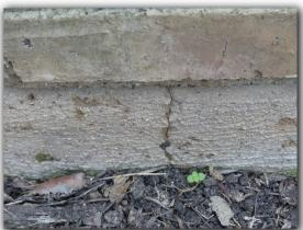
☑ Foundation slab corners have been sheared off (corner pop). This is a common condition in slab on grade foundations and should be repaired. Repairing corner pops is recommended to prevent moisture and wood destroying insect penetration.
