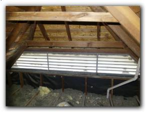
☑ Soffit vents were observed to be dirty, blocked by insulation or debris. Clogged soffit vents are an indication of inadequate attic ventilation and should be repaired as needed.
