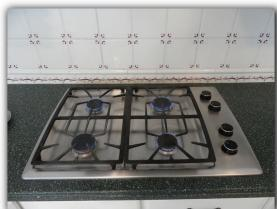
$\ensuremath{\square}$  Missing and or damaged control knob indicators on the range/cooktop/oven should be repaired or replaced.
