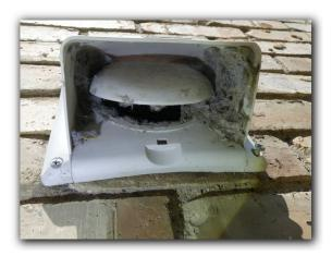
☑ The dryer vent flapper was stuck in open position and was in need of repair or replacement. Dryer vent flappers that are stuck in the open position may allow moisture, insect and unwanted wildlife intrusion.
