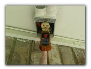
☑ One or more 220V electrical receptacle was observed to be without electric power. The reason for a lack of electric power at 220V electrical receptacles should be determined and repaired as needed by a certified, licensed electrical specialist.
