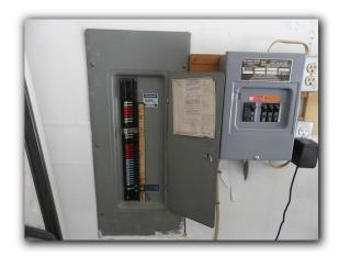
☑ The electric service panel did not have adequate clearance or accessibility. Adequate clearance and accessibility of 36" around the electric service panel should be maintained for reasons of safety.
