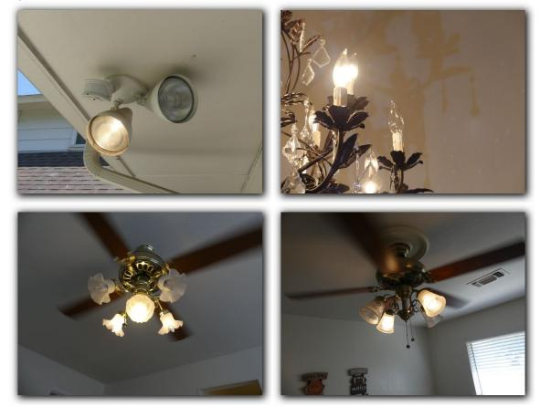
$\ensuremath{\square}$  Exterior light fixtures should be sealed at the wall to prevent water intrusion for reasons of SAFETY.
