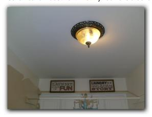
☑ Current building standards require that all bathrooms have installed a mechanical exhaust vent or an operable window to remove moisture from the air. Lack of an operable window or a mechanical exhaust vent in bathrooms is a deficiency and should be repaired.
