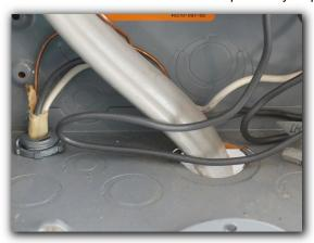
☑ The primary ground rods and conductors were not visible or were missing. It was common in older construction for the primary electrical ground to be connected to foundation metal components or other locations that may not be visible. Under current electrical standards, the primary ground rods and conductors should be visible. It is recommended that the electrical grounding conductor installation be further evaluated by a qualified electrical specialist.
