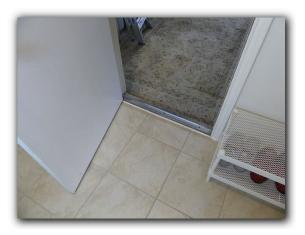
☑ The garage entry door was observed to be a non-fire rated door. Under current building standards, the entry door between the garage and the living area should have a minimum of a 20-minute fire block rating for improved FIRE SAFETY. Lack of a fire rated garage entry door is a SAFETY HAZARD.
