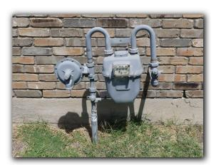
☑ Older style gas valves require a tool to operate. Under current building standards, gas valves should be operable by hand for reasons of safety.
