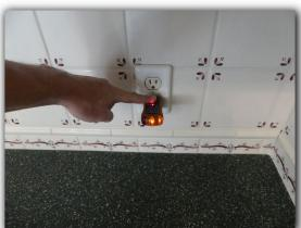
☑ The food waste disposer electrical receptacle was observed to lack ground fault circuit interrupter (GFCI) device protection. According to the 2014 NEC electrical standards, food waste disposer electrical receptacles should be GFCI protected. Lack of GFCI protection in required locations is a SAFETY HAZARD.
