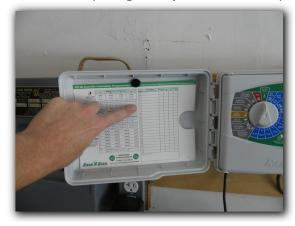
☑ The landscape irrigation system lacks a sensor to disable the system in the event of rain or freezing temperatures.
