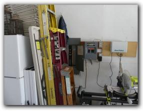
$\ensuremath{\square}$  The electric service panel breaker use was not labeled. Each electric service panel breaker should be adequately labeled as to what appliance or circuit it serves.
