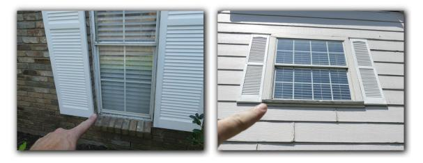
☑ Windows were observed to be missing cap flashing. Missing window flashing should be repaired or replaced as needed.
