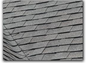
☑ There were indications of impact damage on the roof covering. Impact damaged roof covering shingles may allow further deterioration of the roof covering, deterioration of the roof structure, water penetration or other damage.
