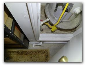
☑ Improper water heating equipment base supports or floors were observed. Improper water heating equipment base supports may not provide adequate support and should be repaired to prevent water heater damage, plumbing damage and water damage.
