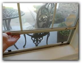
☑ Damaged window screens were observed. Window screens help protect window glass from minor impact damage and prevent insect penetration at the windows. Damaged window screens should be repaired or replaced.
