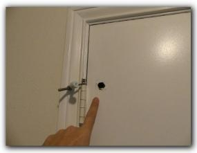
$\ensuremath{\square}$  All interior doors should have door stops installed to prevent damage to adjacent interior wall coverings.
