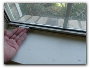
☑ Damaged window lift supports were observed. Damaged window lift supports may not hold windows in the open position and may allow glass or window frame damage. Damaged window lift
