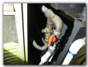
☑ The gas supply flex connector at the heating equipment was observed to be passing through the heating equipment cabinet. Only rigid black gas pipe is allowed to pass through the heating equipment cabinet (appliance wall) (SAFETY HAZARD).
