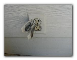
☑ Painted electrical receptacles were observed. Painted electrical receptacles are considered damaged and should be replaced by a certified, licensed electrical specialist for improved safety and performance.
