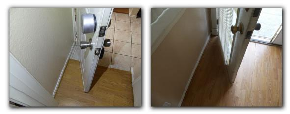
☑ Damaged or missing exterior door weather stripping should be replaced. Missing or damage exterior door weather stripping creates conducive conditions for moisture intrusion and conditioned air loss.
