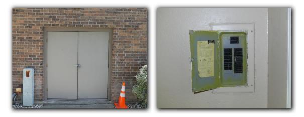
☑ The electric service panel breaker use was not labeled. Each electric service panel breaker should be adequately labeled as to what appliance or circuit it serves.
