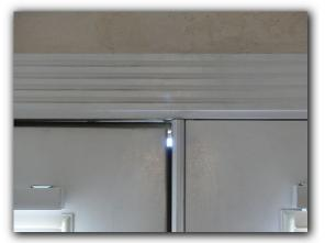
☑ Exterior doors that rub, stick or hit door frames were observed. Exterior doors that stick, rub, hit the door frame or do not perform as intended are indications of movement, settlement or other defects. The cause of exterior doors that rub, stick or hit door frames should be determined and repaired as needed.
