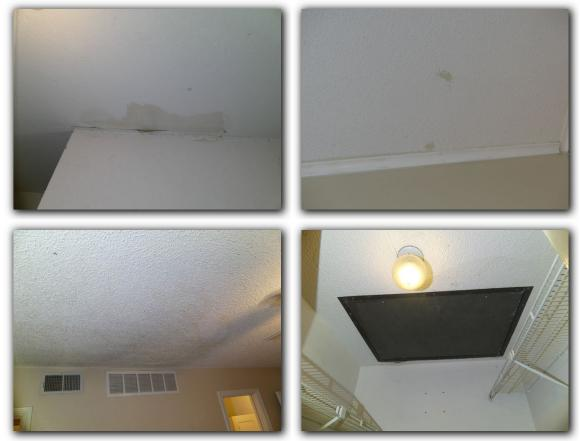
☑ At least one interior ceiling crack was observed which is an indication of structural settling,
