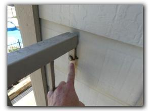
☑ The stairway risers were open and were observed to be a SAFETY HAZARD. Under current building standards, stairway risers should not allow passage of any object greater than 4".
