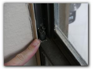
☑ Damaged, missing or inoperative window lock(s) were observed. Damaged, missing or inoperative window locks are a SAFETY HAZARD and should be repaired prior to occupancy.
