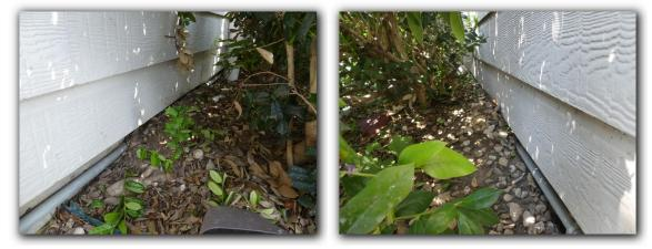
☑ There is a subsurface or below grade drainage system installed. The inspector has no way of knowing if below grade drainage systems are performing as intended. The inspector recommends that the below grade drainage system be monitored for performance.
