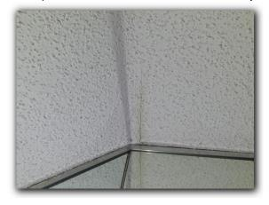
$\square$  Water stains or water damage was observed at the ceiling drywall, texture and paint. The cause of the water staining or water damage should be determined and repaired as needed.
